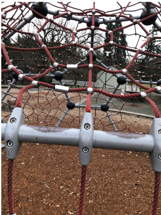
Exposed metal on posts (high usage/age)
