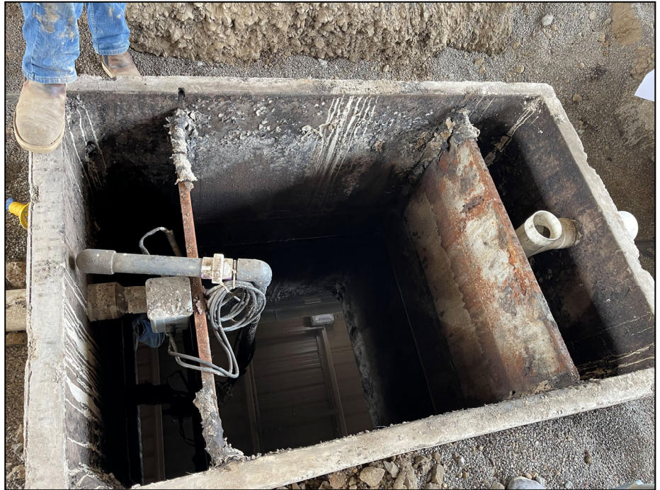
Oil separator vault—bad, removed from service
