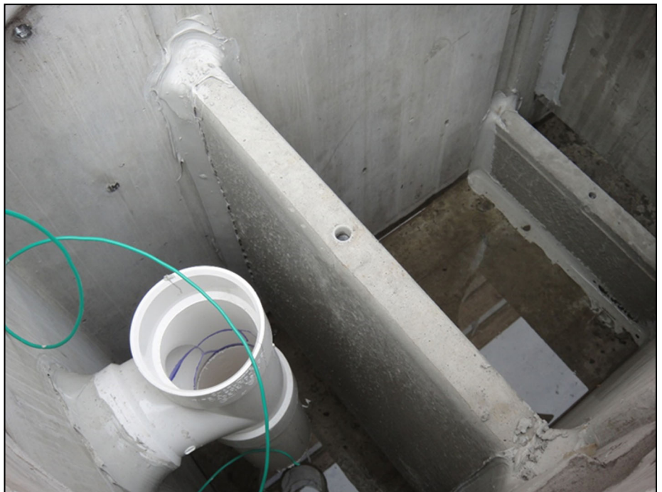
Oil separator vault—new replacement
