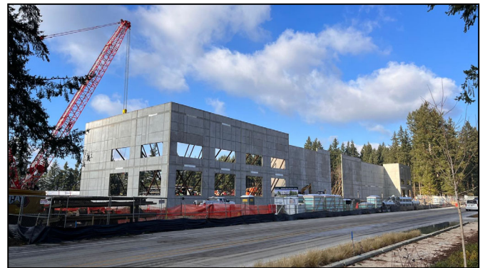
New concrete wall panels being installed at the Grahams Ferry Industrial Center on Garden Acres Road
