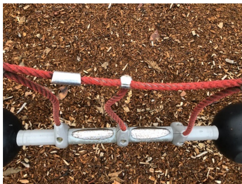
Braided cable exposed (high usage)
