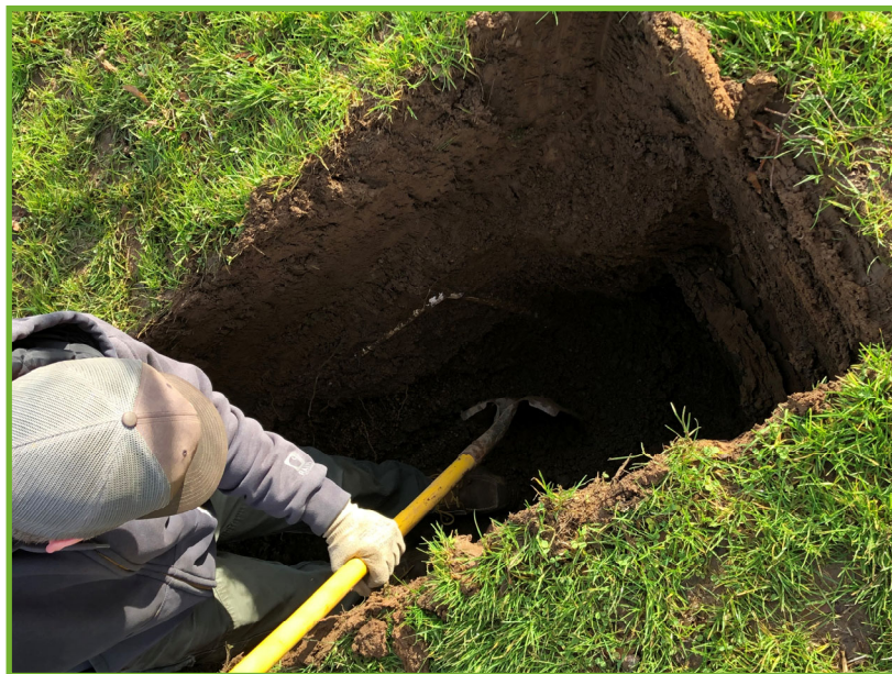
Digging down to the service line
