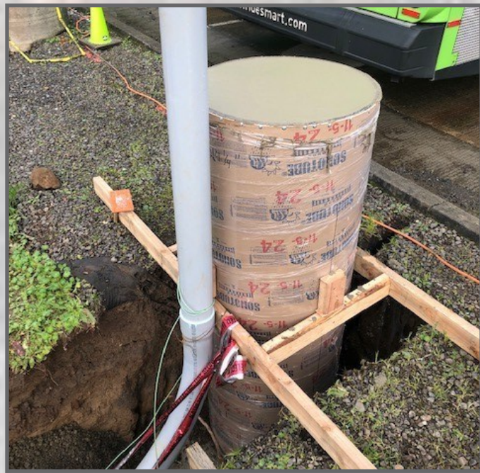
Forming and mockup of a fuel dispensing post
