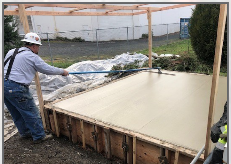
Finishing concrete for compressor installation location.
