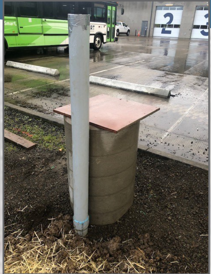
Completed fuel dispensing post support structure, awaiting hardware installation.
