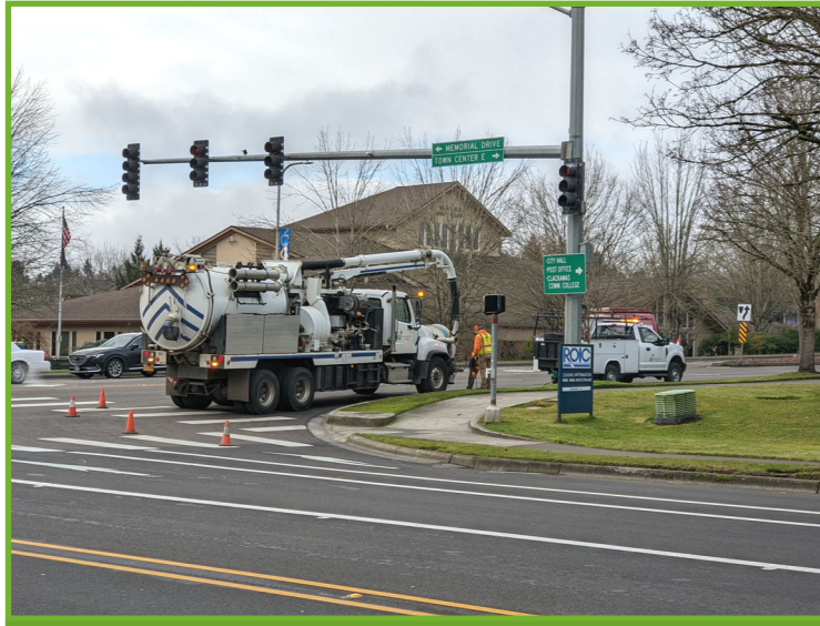
Stormwater Crew at work!
