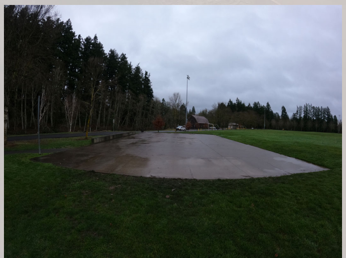
Remaining Concrete Pad
