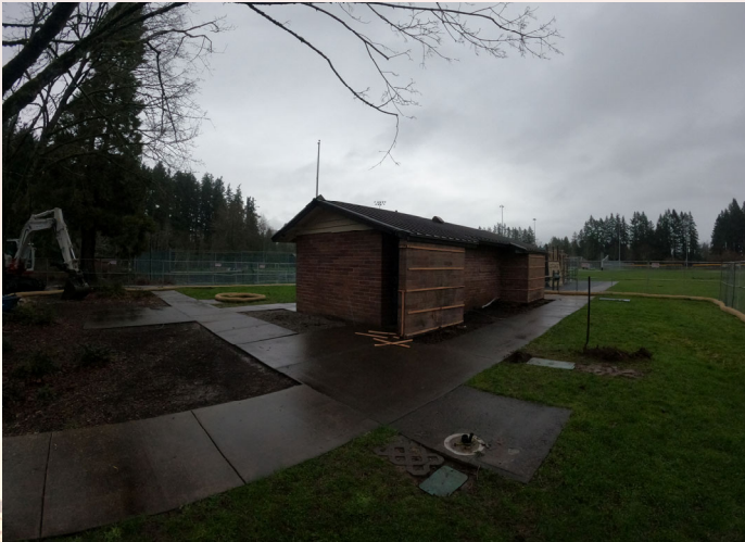
Restroom Demo Begins
