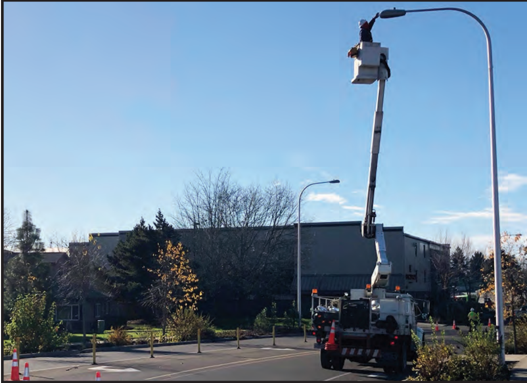
LED streetlight conversion project - light installation.
