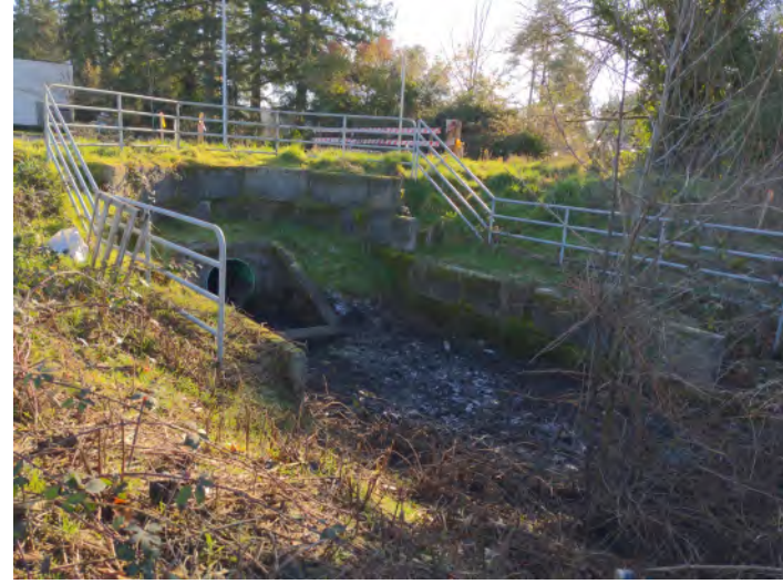
Photo 2. Existing stormwater facility in the southern portion of the site.
