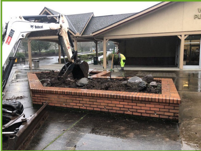
Working at the Library entrance
