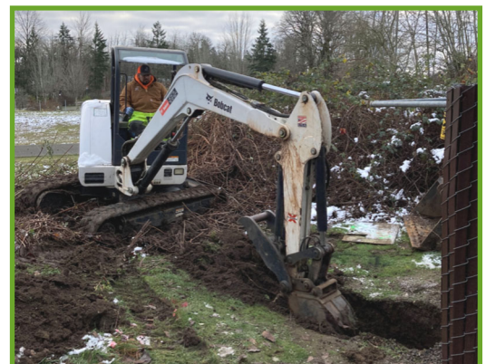
Excavating the sinkhole
