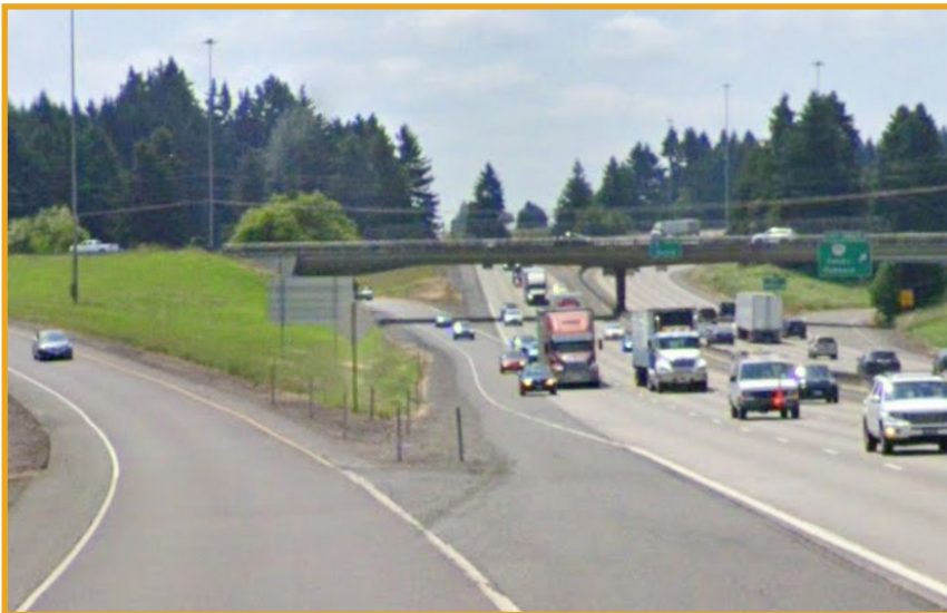
Above: Short merging distance between the OR 551 Canby-Hubbard entrance ramp and Charbonneau entrance ramp and heavy freight use cause safety conflicts resulting in a top 10% SPIS site.
