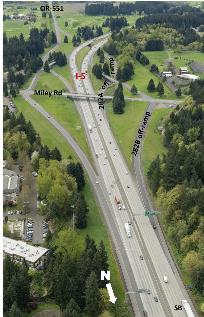
FIGURE 6. I-5 and the Charbonneau District (Exit 282B) and Canby-Hubbard (Exit 282A) interchanges.
