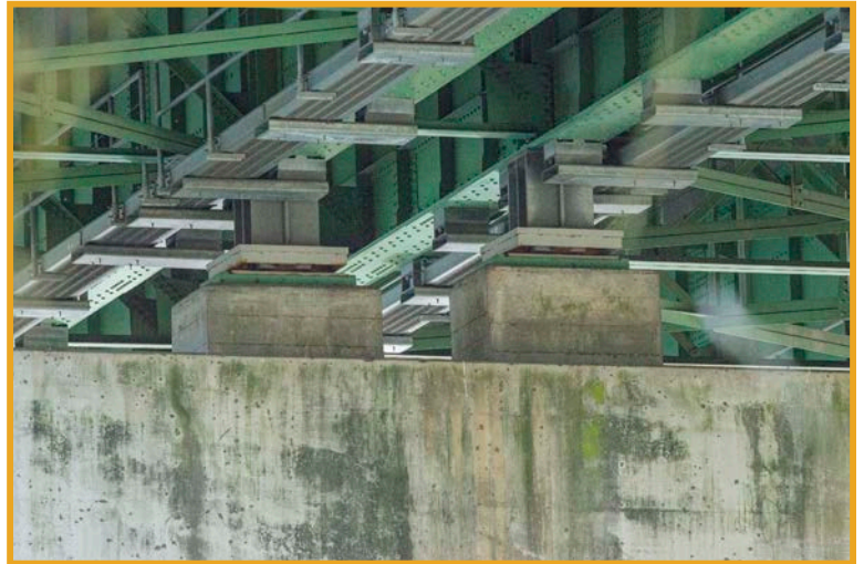
Above: Existing railing and pier supports of the Boone Bridge.
