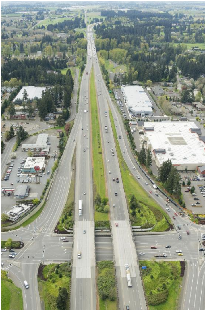
FIGURE 3. Aerial photo of the study area, as viewed from above the I-5: Wilsonville Road interchange looking south along I-5.
