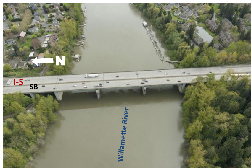
FIGURE 5. I-5 Boone Bridge over the Willamette River.
