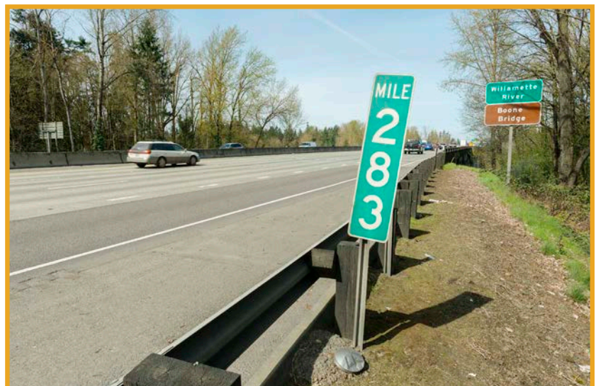
Right: I-5 northbound mile marker 283 on the south end of the Boone Bridge.
