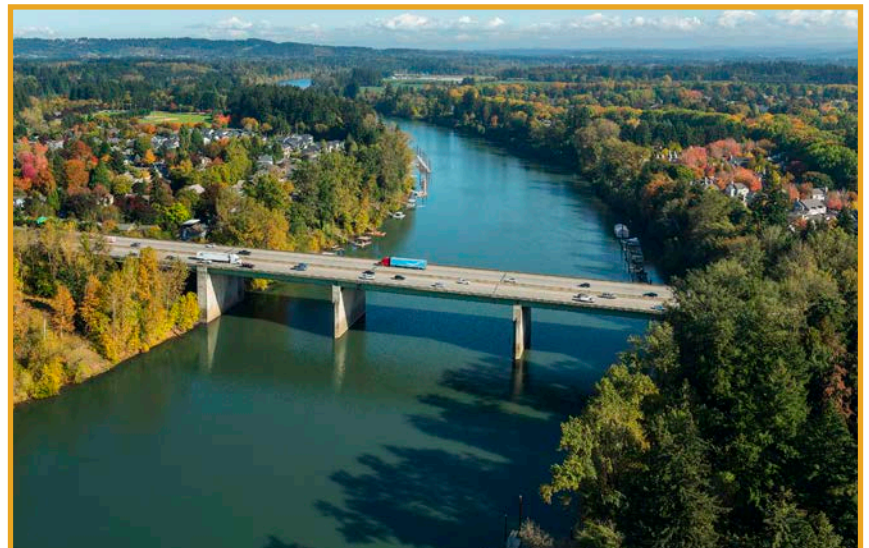
Above: The I-5 Boone Bridge.
