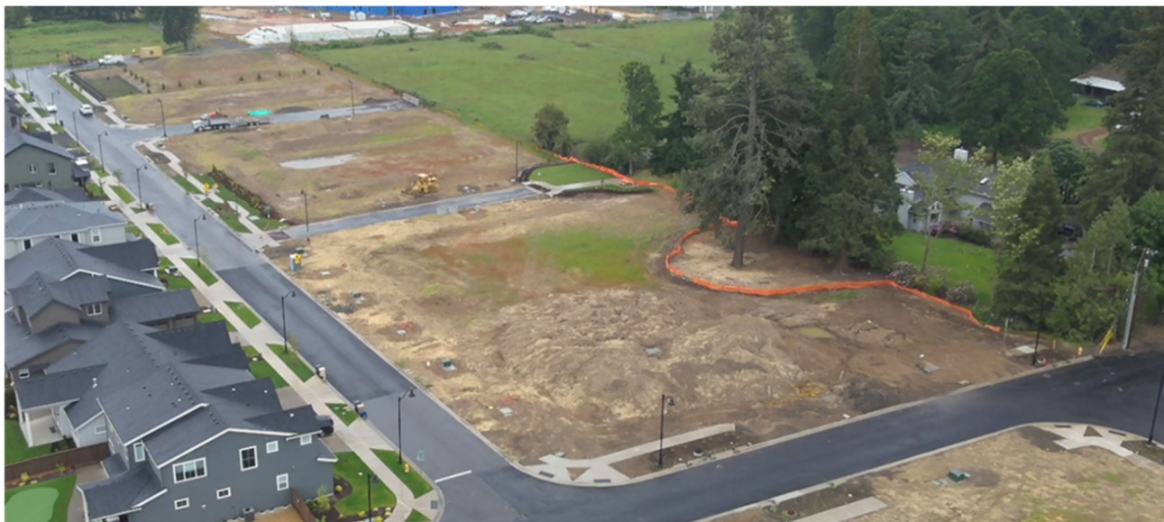
Aerial view of the Frog Pond Estates site
