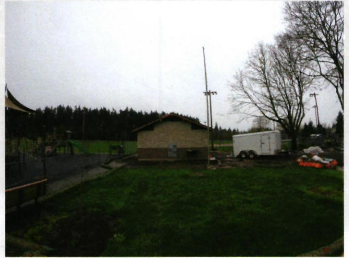
Plumbing Contractor Onsite
