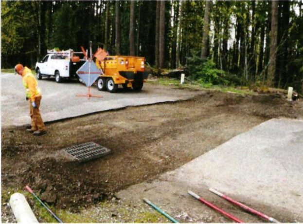
Preparing Base Gravel
