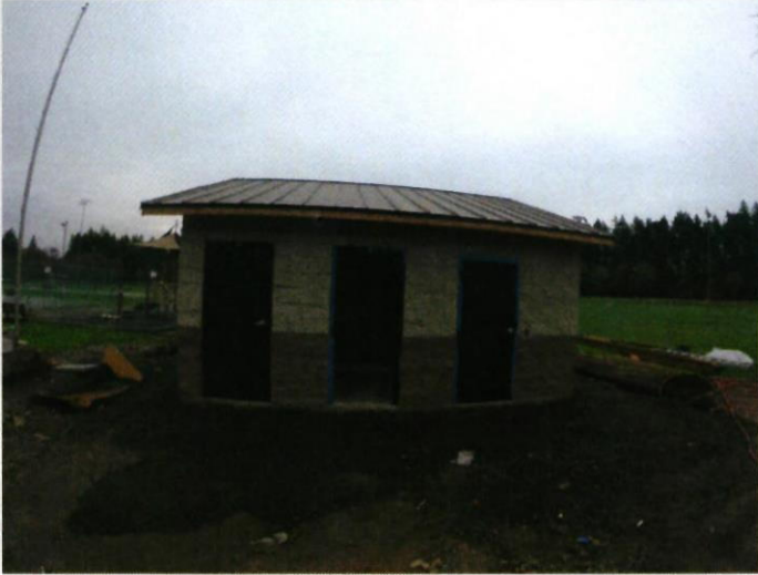
Restroom Awaiting A Sidewalk
