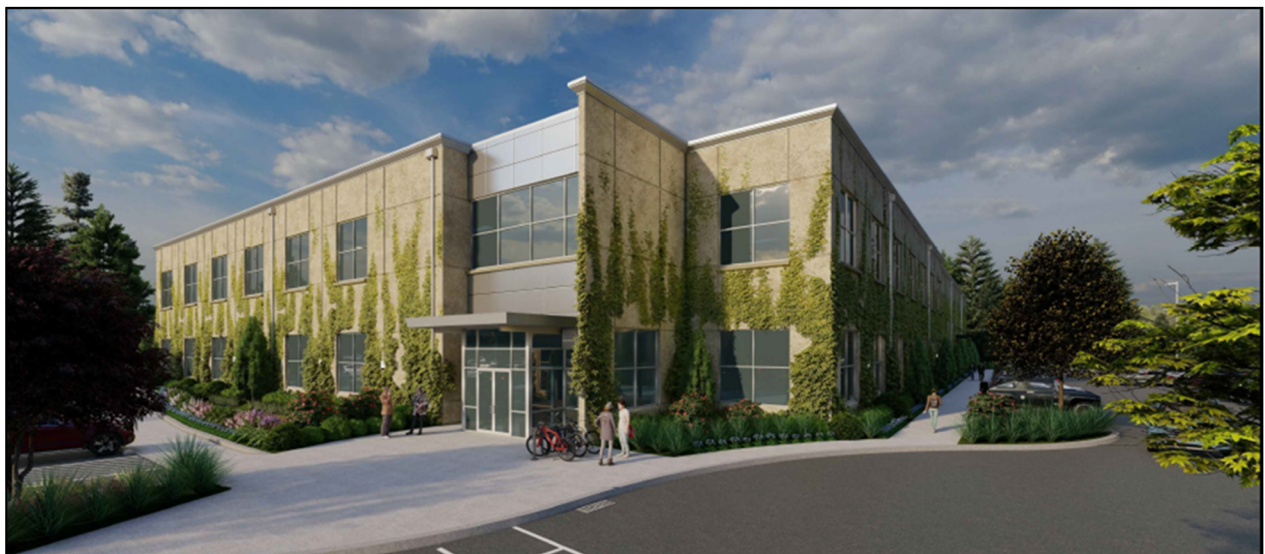
Perspective of Proposed Industrial Building at Kinsman and Boeckman from Boeckman Road
