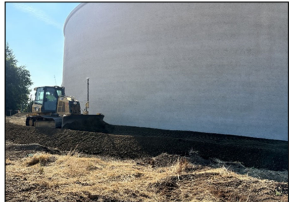
Backfilling around reservoir
