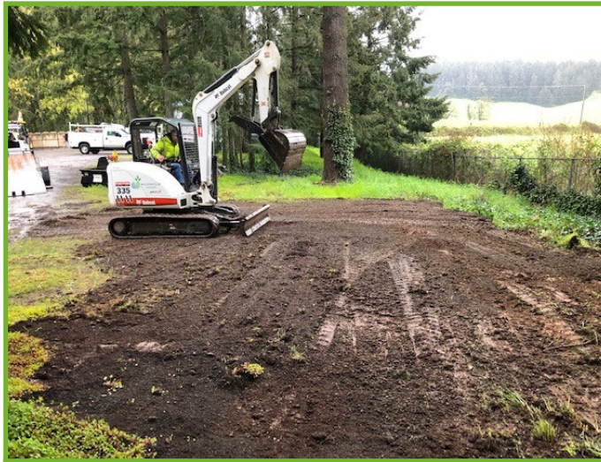
Leveling the site
