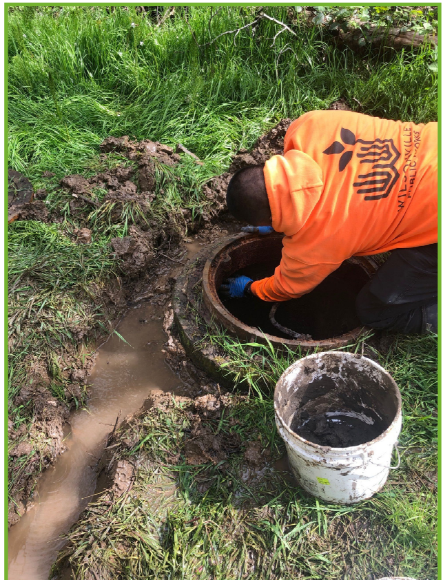
David sealing up the casting
