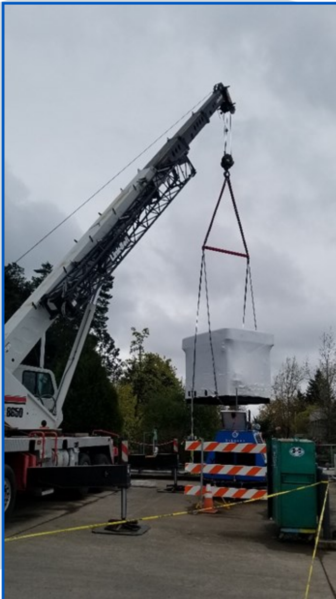
New compressor enclosure being set in place.
