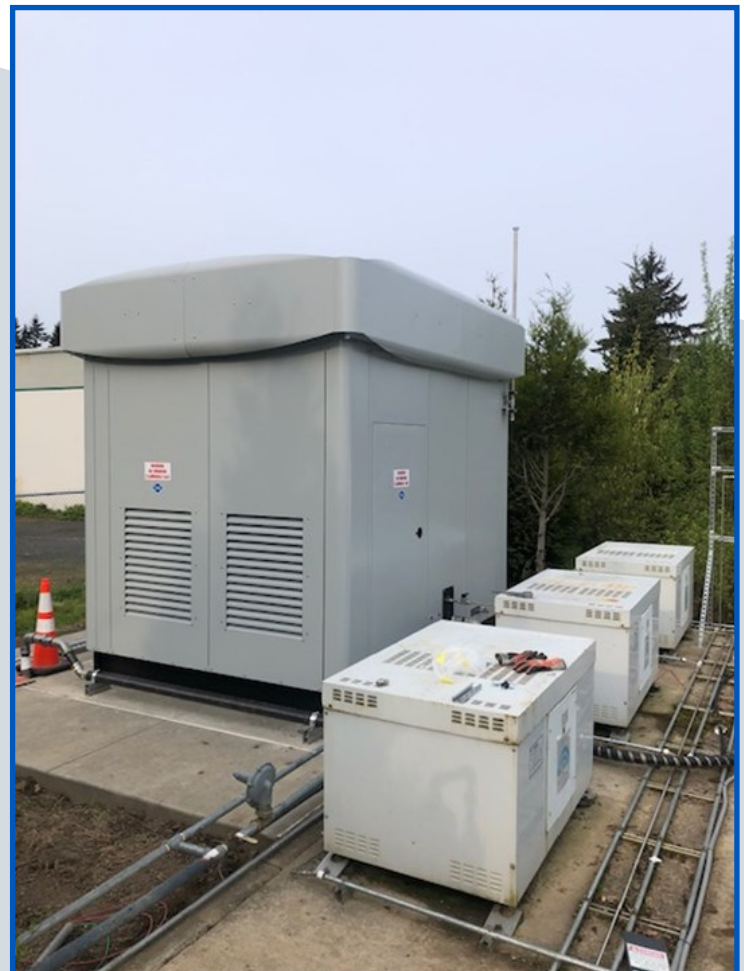
New compressor after installation.
