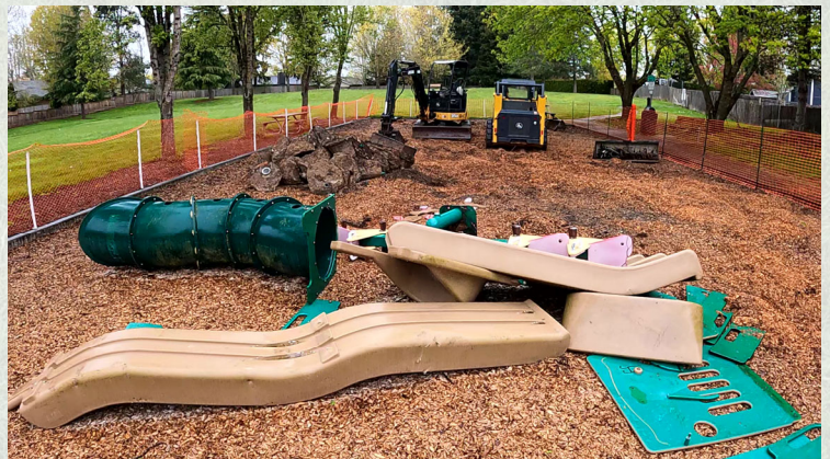
Old Playground Ready for Removal
