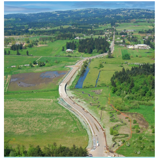
Boeckman Road Construction (2008)
