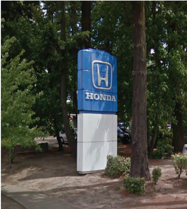
Existing 10x10x20 pylon to be removed and disposed.
