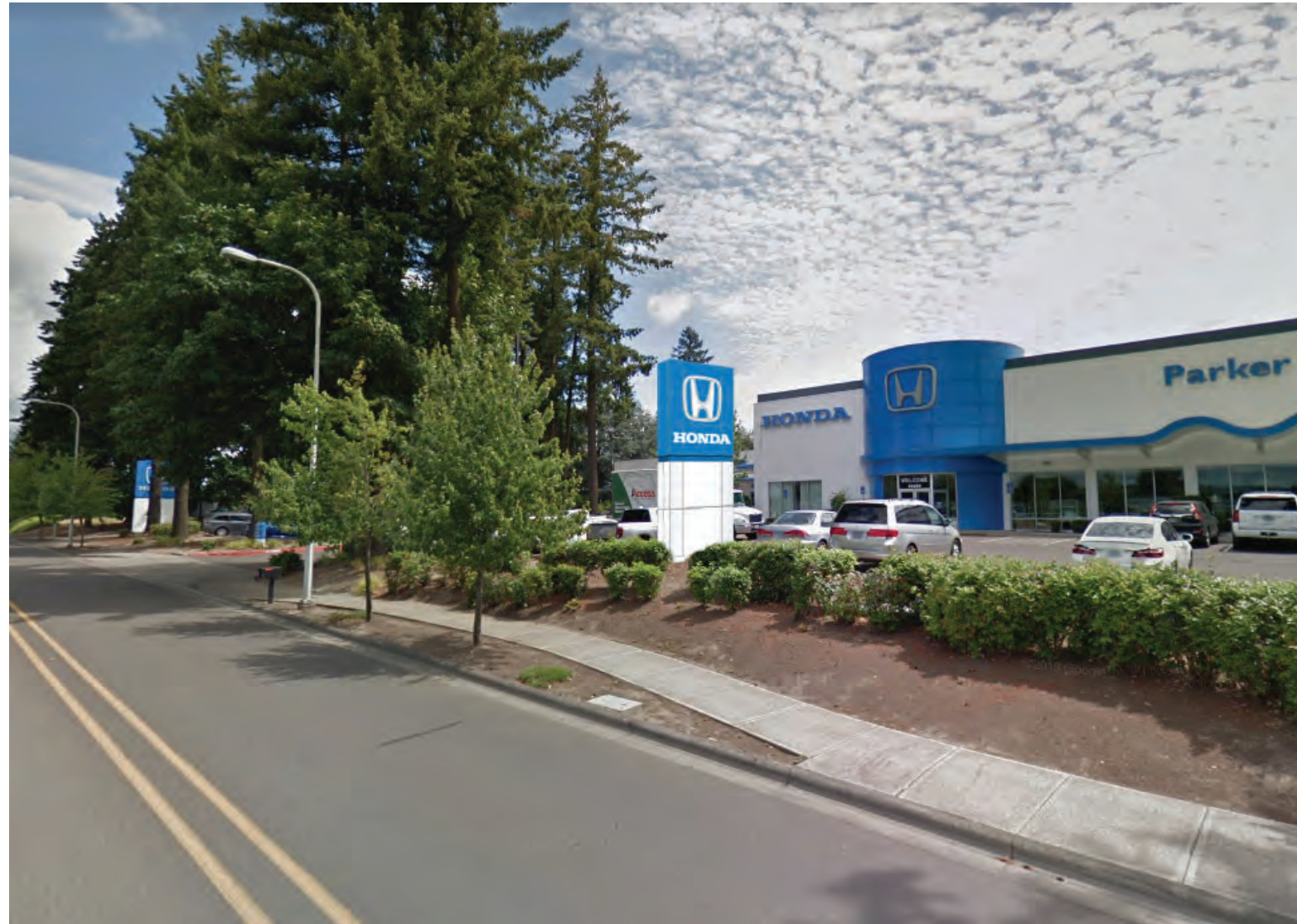
New 8x8x17 pylon installed in new location.
