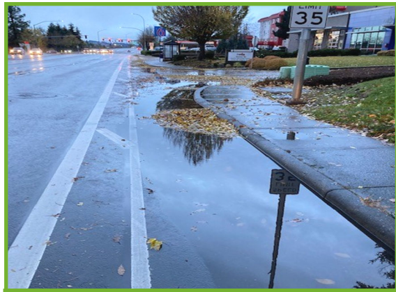
Leaf accumulation causing flooding
