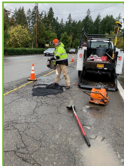
Pothole repair
