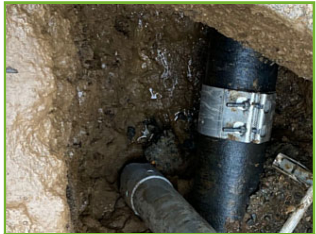
Repair band installed
