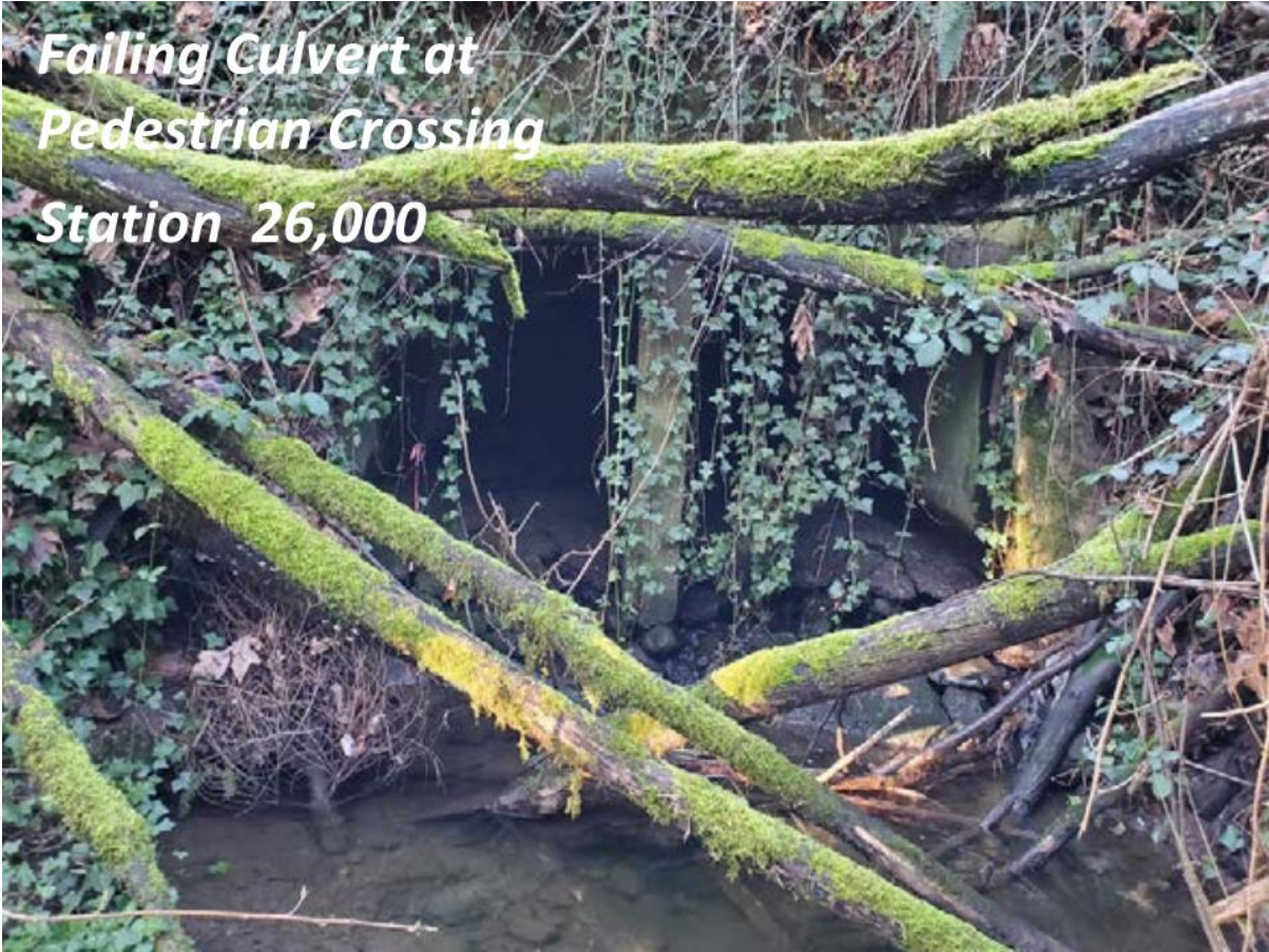
Failing twin 5 ft x 5 ft culverts under pedestrian crossing looking upstream (Source: Geomorphic Stream Assessment, Waterways Consulting, May 2022)
