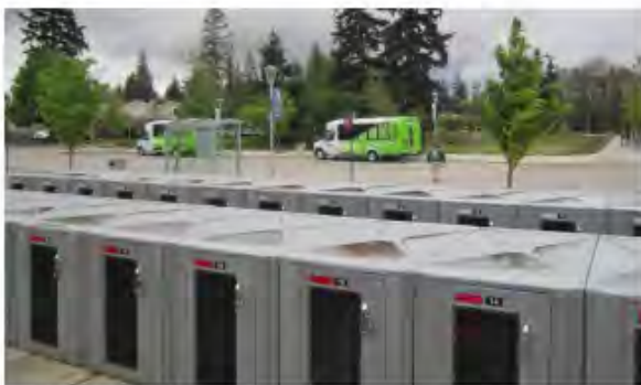
Bike lockers at the SMART Central at Wilsonville Station transit center provide secure storage for transit riders who use their bikes to complete a leg of their trip.
