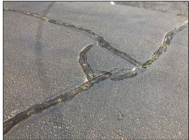
Photo 4: North Parking Bay – Crack Seal closeup
