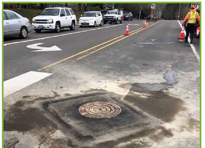
Finished project ready for traffic
