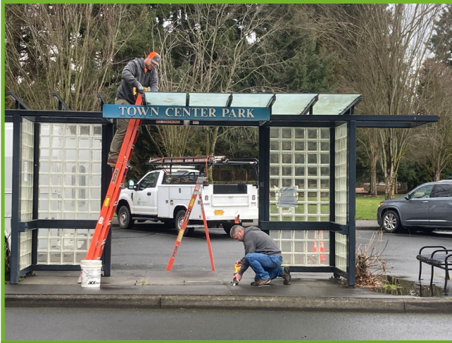
Disassembling the shelter
