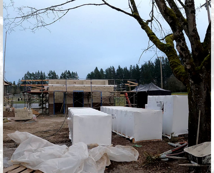
Building Is Roof Ready
