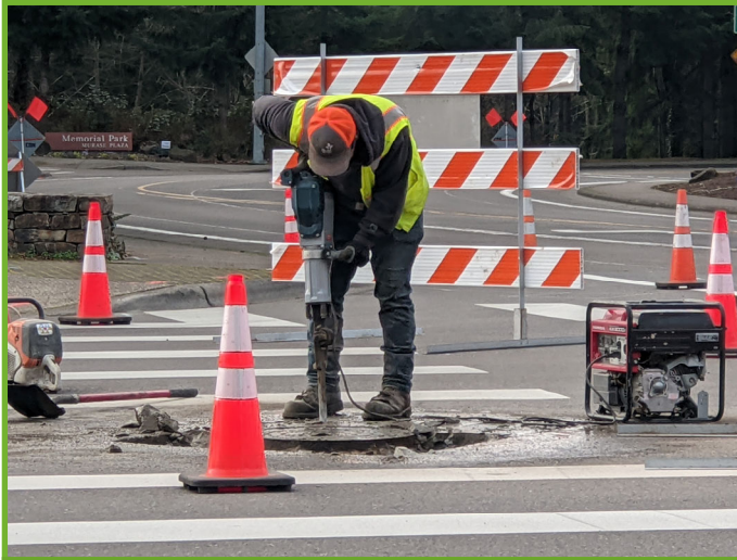
Removing the manhole and concrete collar
