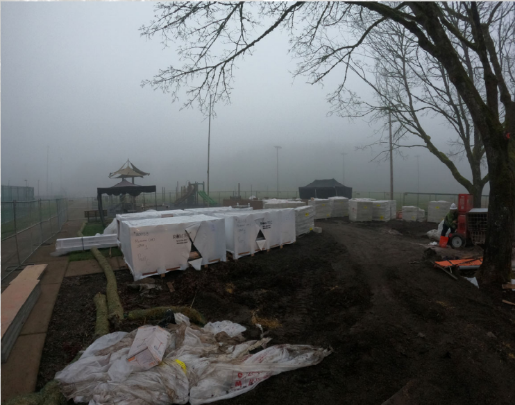
CMU Block Onsite
