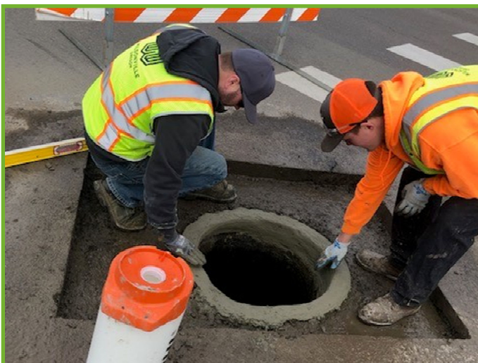
Smoothing the concrete at the top of the manhole
