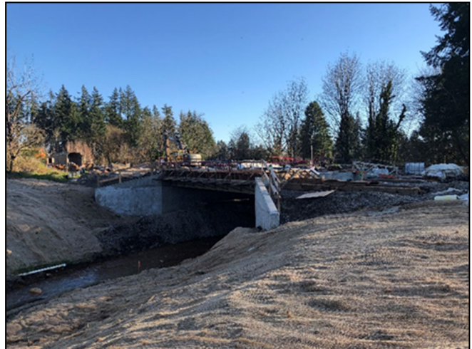
Construction of the 5th Street Bridge
