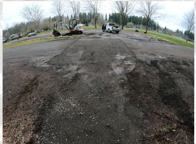
Finished and Awaiting Asphalt
