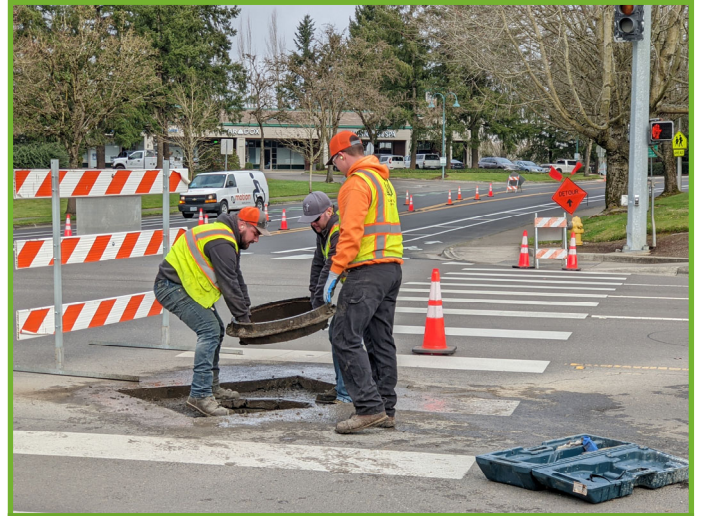
Setting the new metal ring in place
