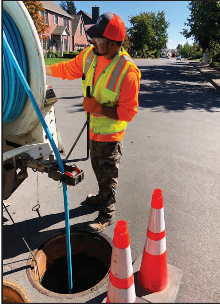
Staff cleaning wastewater pipes throughout the City.
