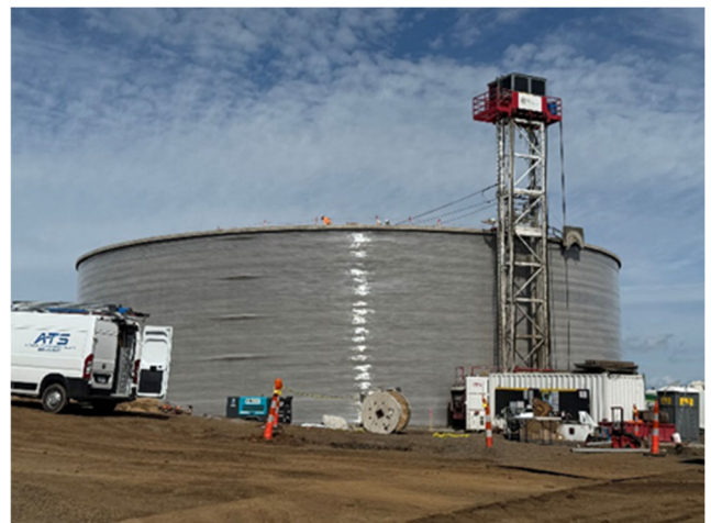
Tank wrapping for concrete cure
