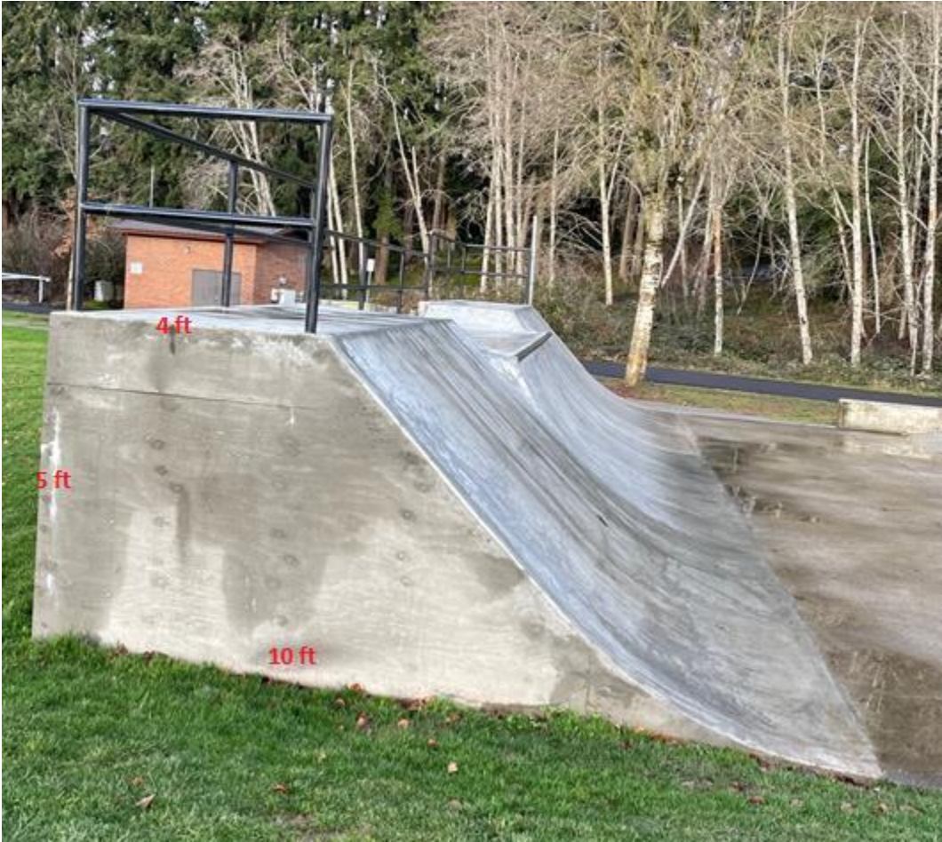
Wall 1 (side of wall 2)
