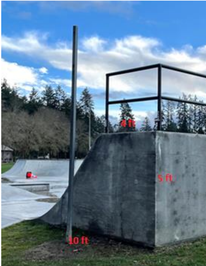
Wall 4 (side of wall 2)
