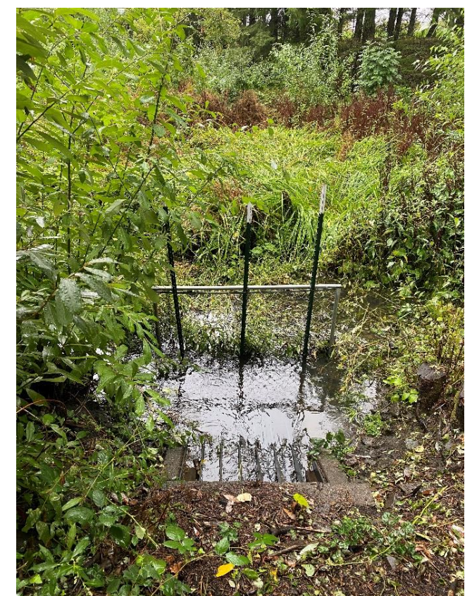
Outlet of pond that functions as the ditch inlet (Sep 2021)
