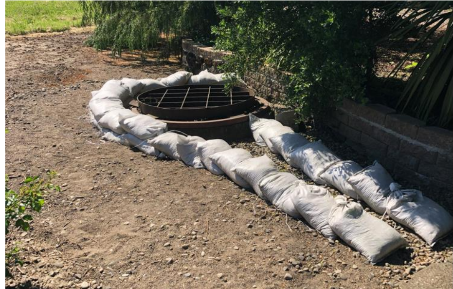
Existing Bubbler Structure (May 2023)
