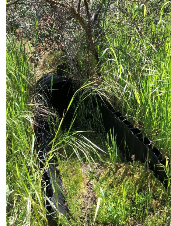
Garden Acres Pond Existing Inflow Pipe (May 2023)
