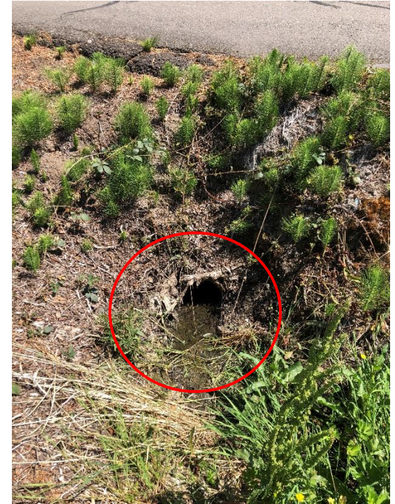
Culvert inlet under Rose Lane (May 2023)
