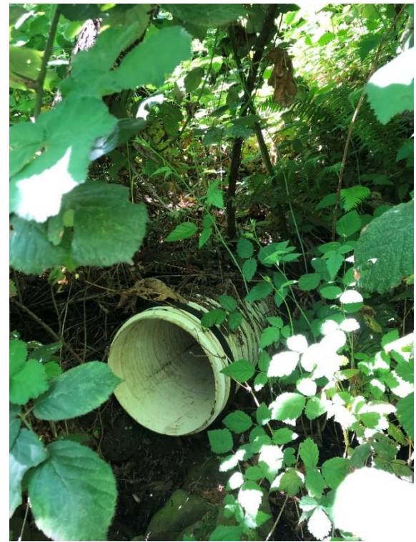
City-owned outfall pipe (May 2023)
