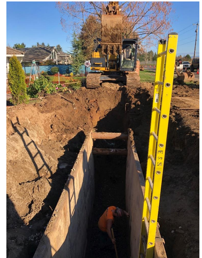
Temporary construction work on sinkhole
