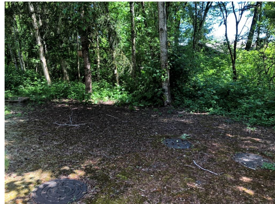
Upstream detention pipes location (May 2023)
