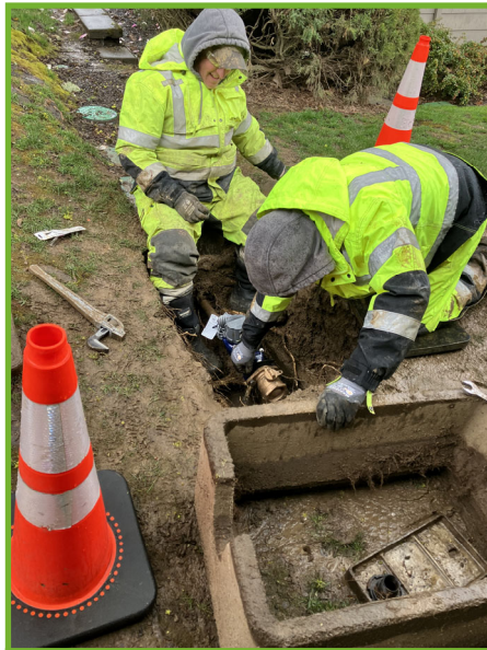
Angle stop repair
