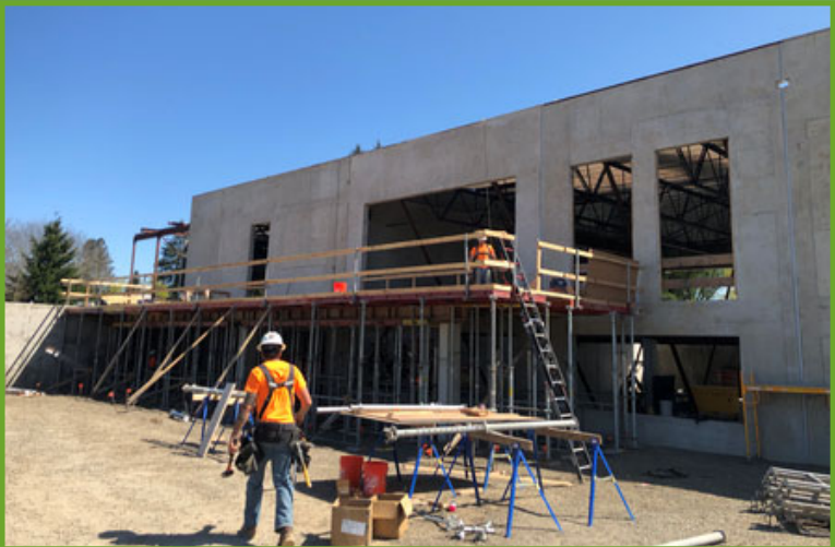
Forming of elevated deck on administration building.
