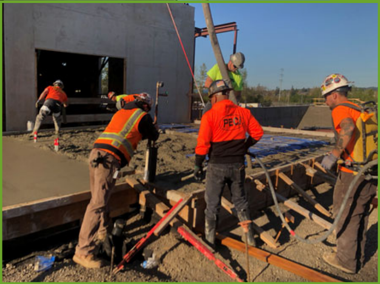
Pouring the slab on grade concrete
