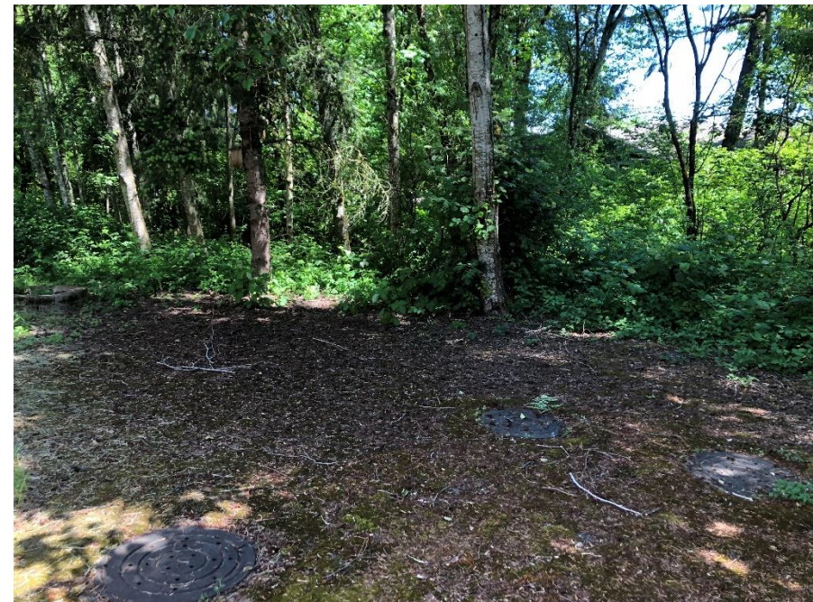
Upstream detention pipes location (May 2023)
