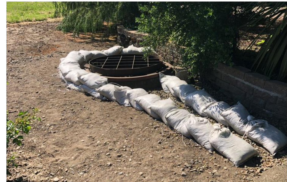
Existing Bubbler Structure (May 2023)
