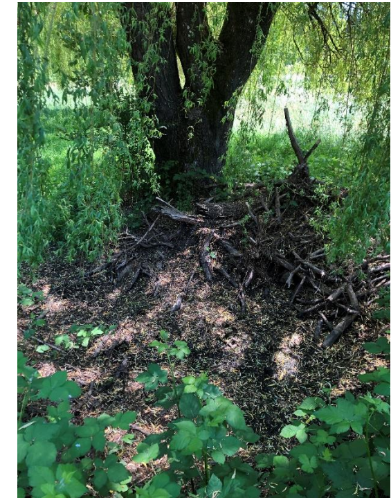
Downstream of culvert, east side of Rose Lane (May 2023)
