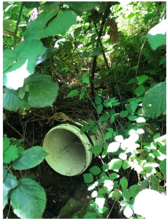
City-owned outfall pipe (May 2023)
