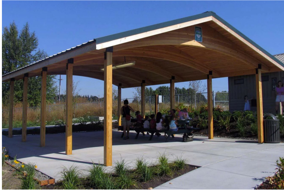
picnic shelter - Western Wood Structures treated Douglas fir, powdercoated steel (dark green), standing seam metal roof (dark green)
