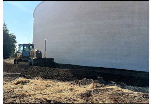
Backfilling around reservoir
