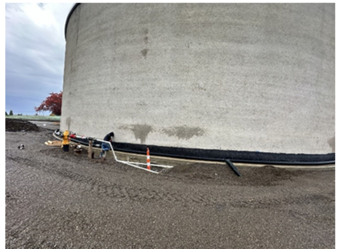
Waterproofing the tank exterior base
