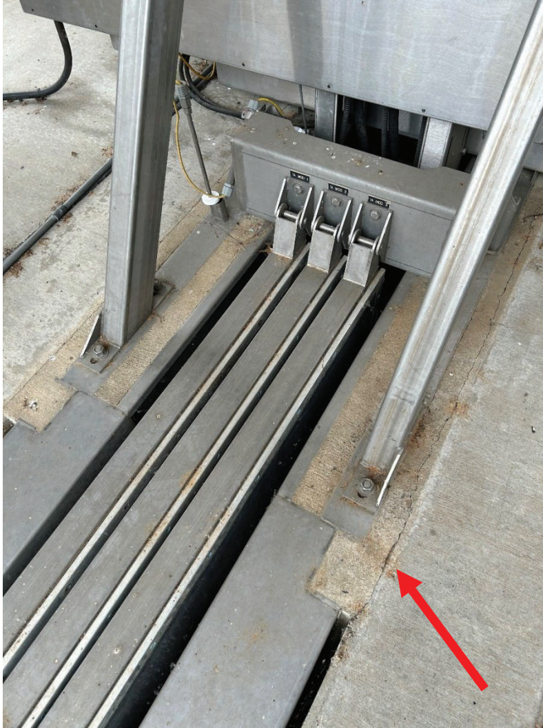
Figure 3-6. Grout-channel interface in the area of the TrojanUV4000
