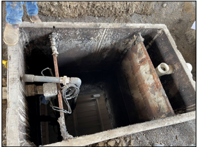
Oil separator vault—bad, removed from service
