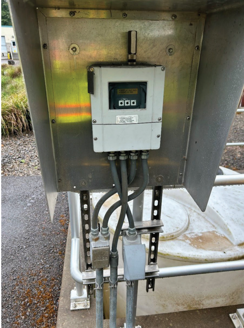
Figure 3-7. Flow meter display
