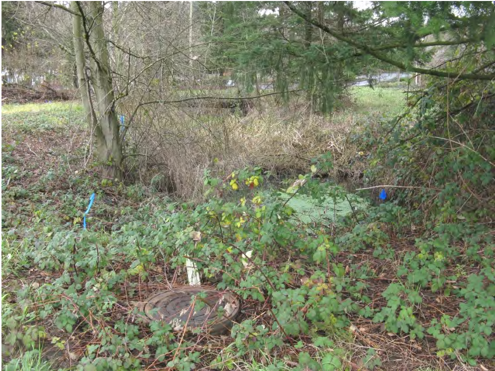
Photo C: Looks east into Wetland B near culvert feeding into Wetland Ditch 1.
