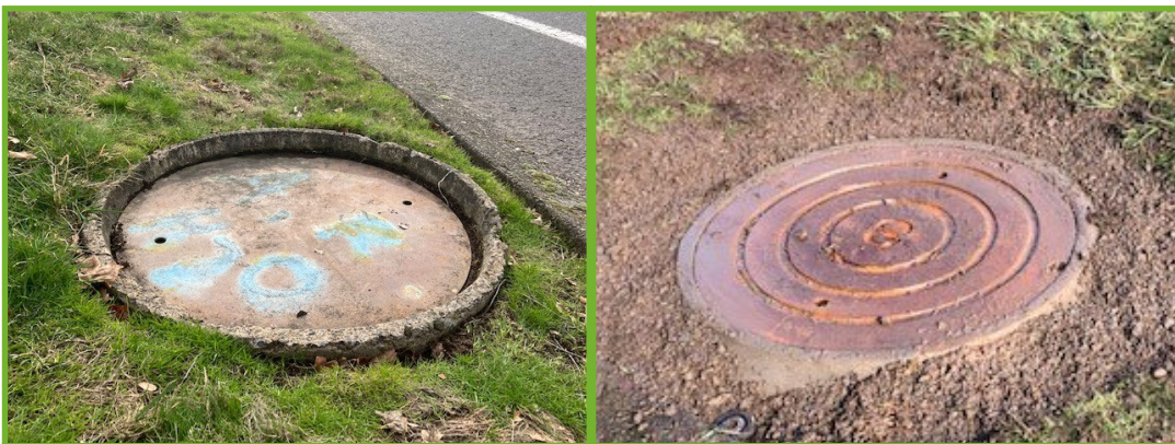
Manhole Repairs—Before and After
