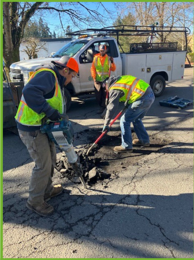
Cutting out the old surface
