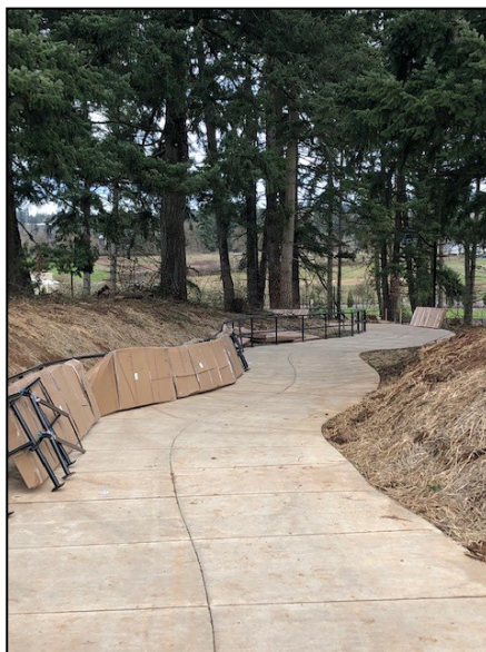
ADA railing being installed.
