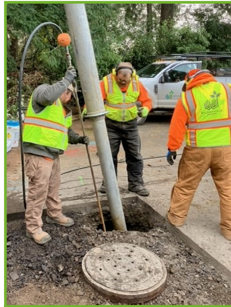
Vactoring a sinkhole
