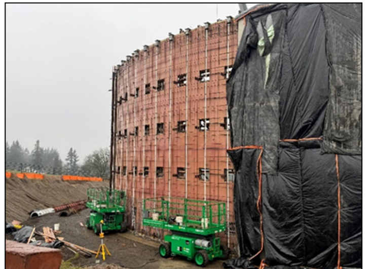
Reservoir wall forms prior to pour.
