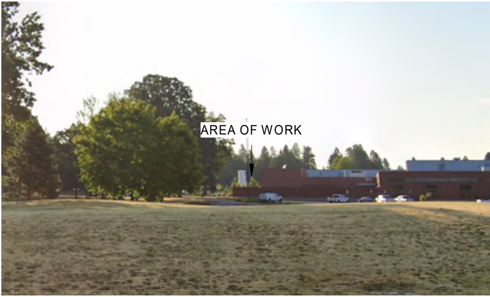
VIEW FROM STREET - 2 AREA OF WORK IS OBSCURED BY TREES.
