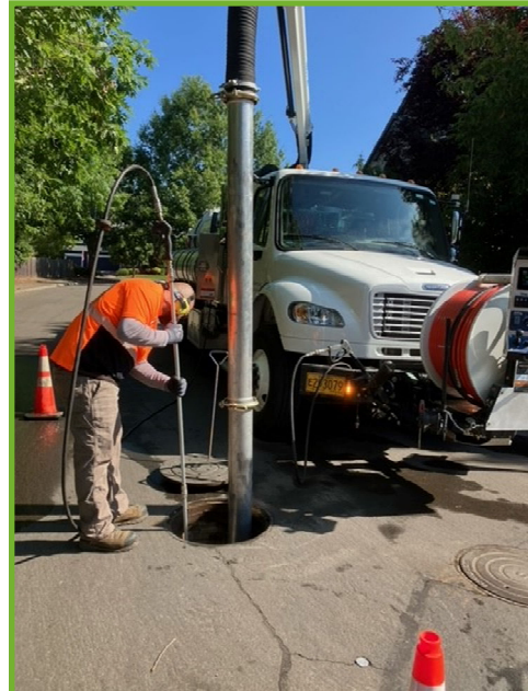
Cleaning water quality manhole
