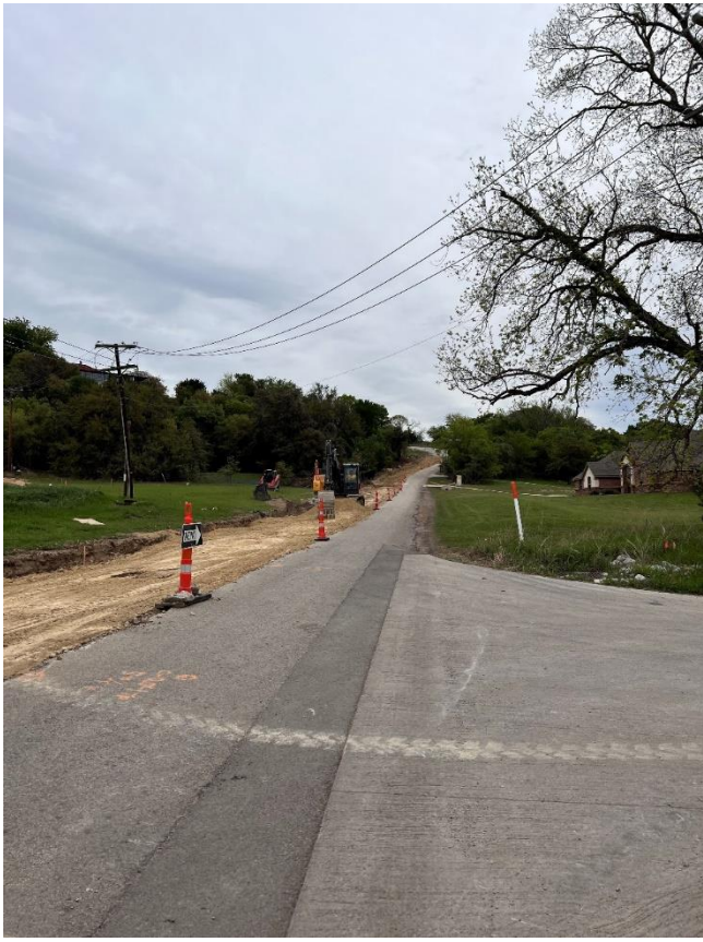
King's Gate Road looking north
