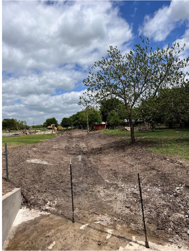
Channel B looking east
