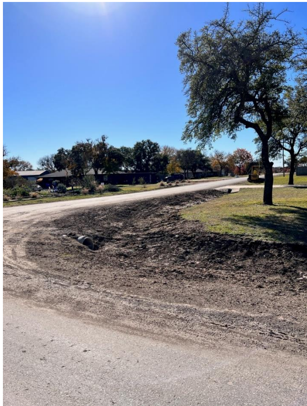
Channel B-2 looking southeast
