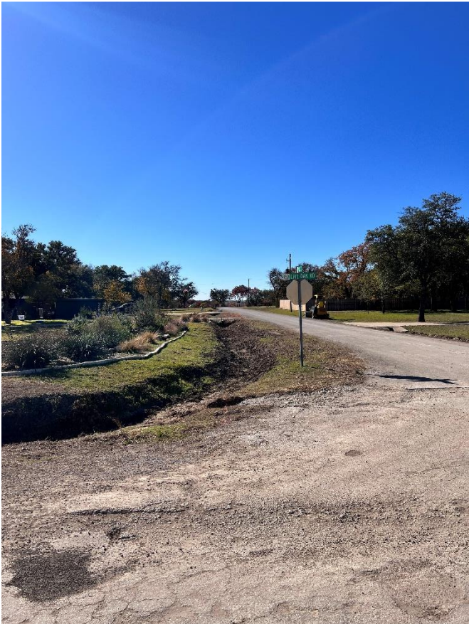
Channel B-1 looking south
