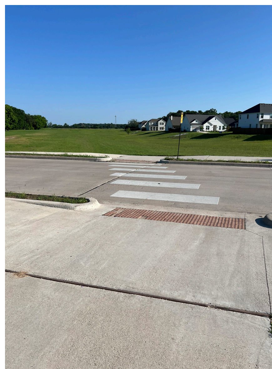
⑪ EXISTING CROSSWALK & RAMPS
