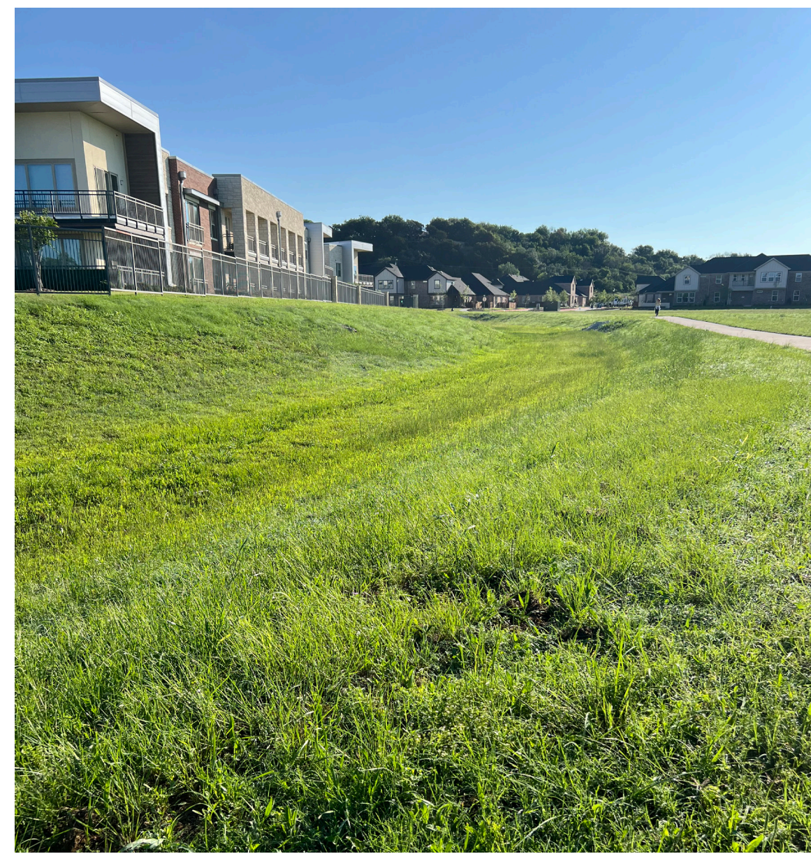
③ EXISTING DRAINAGE SWALE
