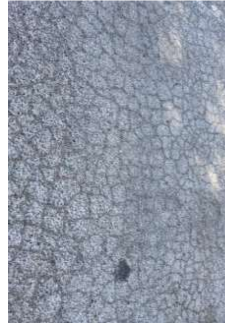
Alligator Cracks
