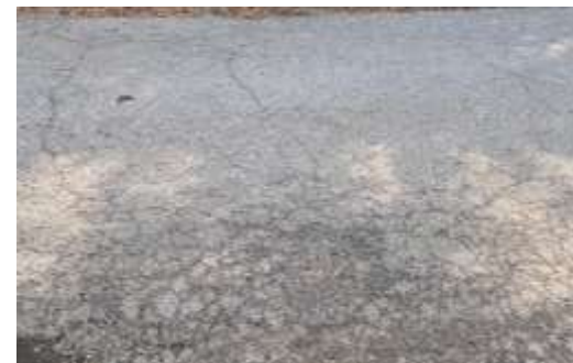
Block cracks
