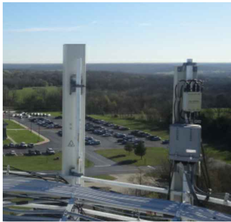
5 EXISTING BETA SECTOR RRU AND RAYCAP LOCATION N.T.S.
