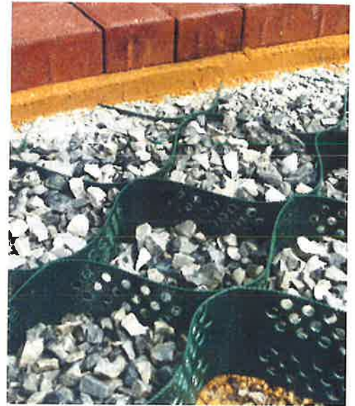
Fig. 2.7 Brick and gravel stabilizer system
