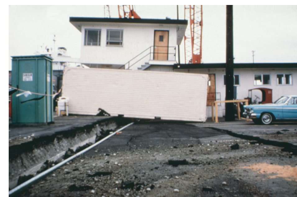
Liquefaction during the 1965 SoTac earthquake caused both lateral and vertical movement of the ground in the Port of Seattle. Cargo cranes such as the one in the background are vulnerable to liquefaction-induced ground displacement. Lateral spreading such as this can cause severe damage to both above-ground structures and underground utilities. Photo courtesy of the Karl V. Steinbrugge Collection, Earthquake Engineering Research Center [ http://misc.berkeley.edu/visual_resources/steinbrugge_collection.html ].
