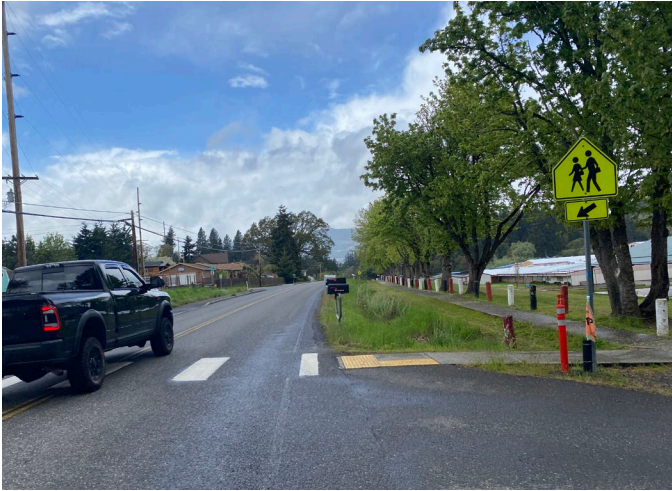
High visibility crosswalk with signage on NW Loop Road near Henkle Middle School.
