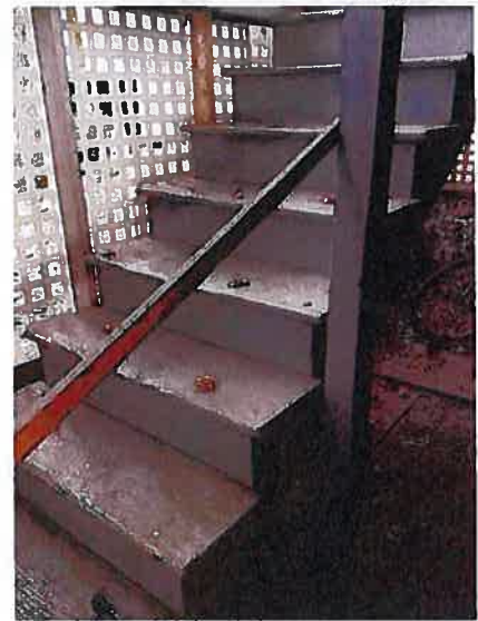
Rear lower S Side stairs
