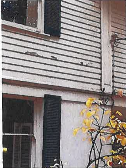
West Side SW bedroom wall
