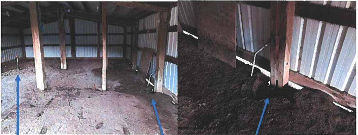
Metal outdoor water hydrant
