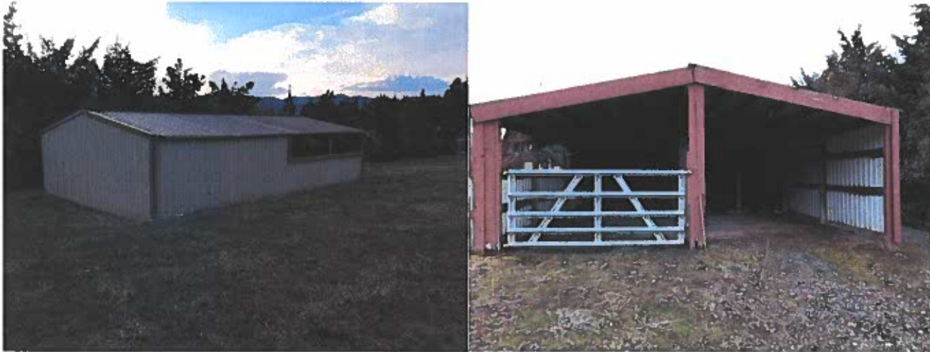
Barn outbuilding where the broken waterline occurred.
