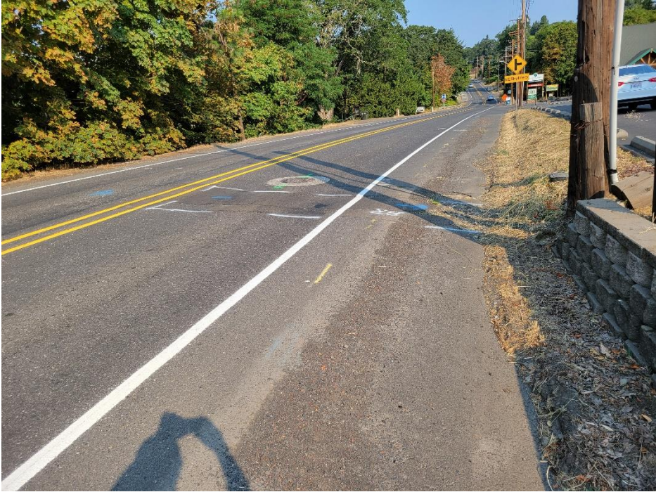
Photograph 7: 1000 E. Jewett Service Line
