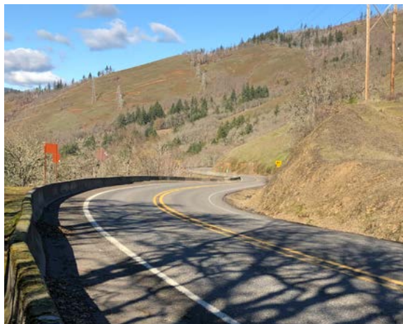
Possible Alignment on SR 141
