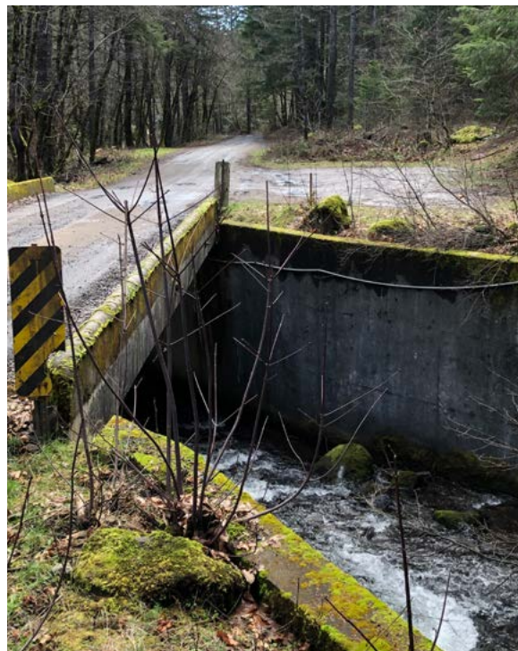
Buck Creek Bridge
