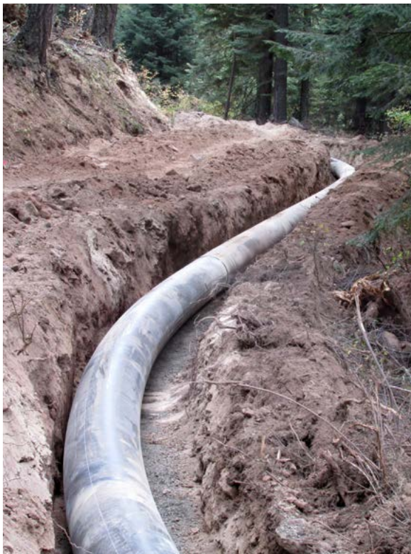
24-Inch Pipeline Installation, City of Cove, OR
