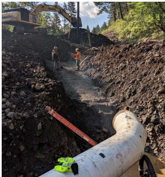
30-inch Waterline Installation, City of Walla Walla
