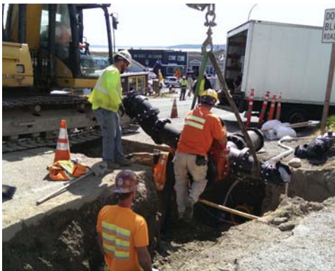
King County Water District 54 – 223 rd Waterline
