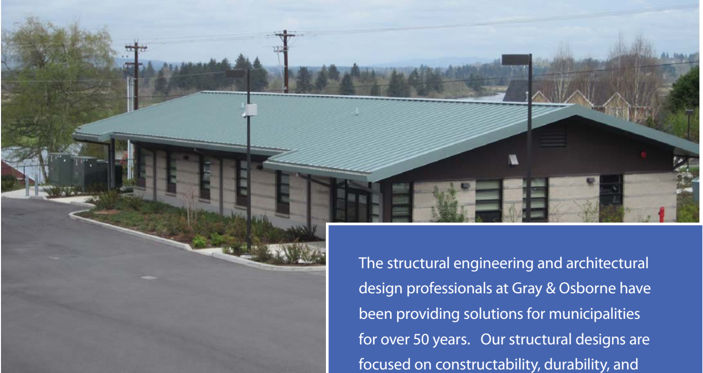
Lake Stevens Sewer District – Wastewater Treatment Facility Administrative Building
