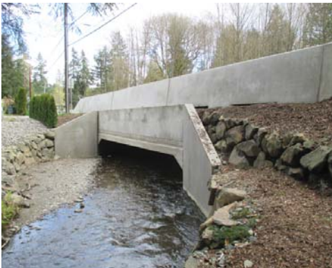
Lake Forest Park – NE 178 th Street Culvert Replacement
