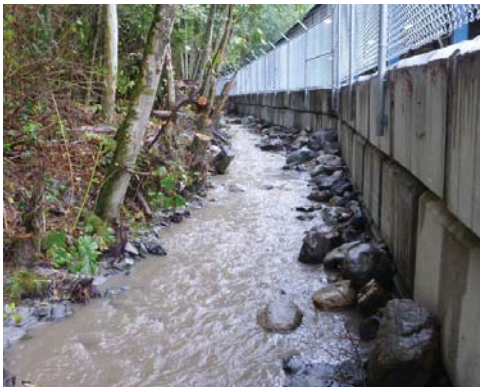
Mukilteo Water & Wastewater District – Emergency Wall Repair
