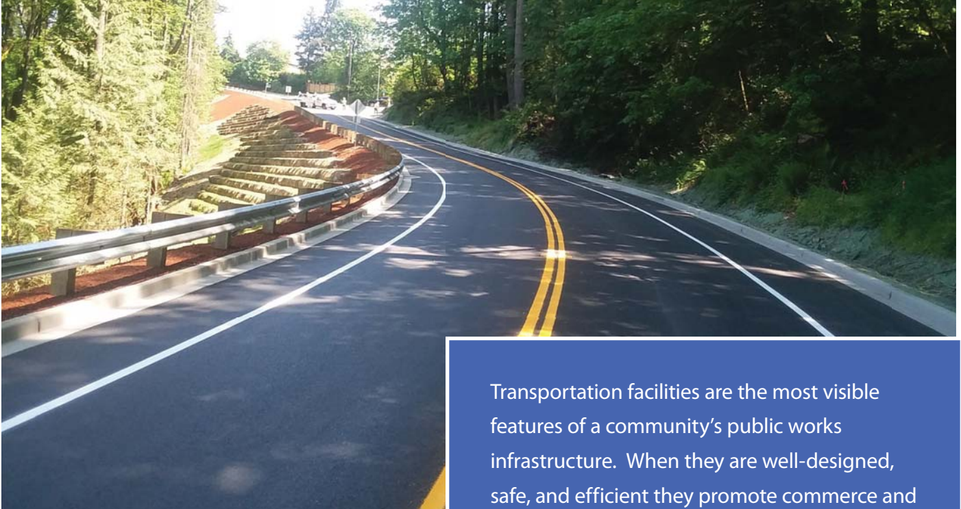
Sammamish – 212 th Way SE Improvements
