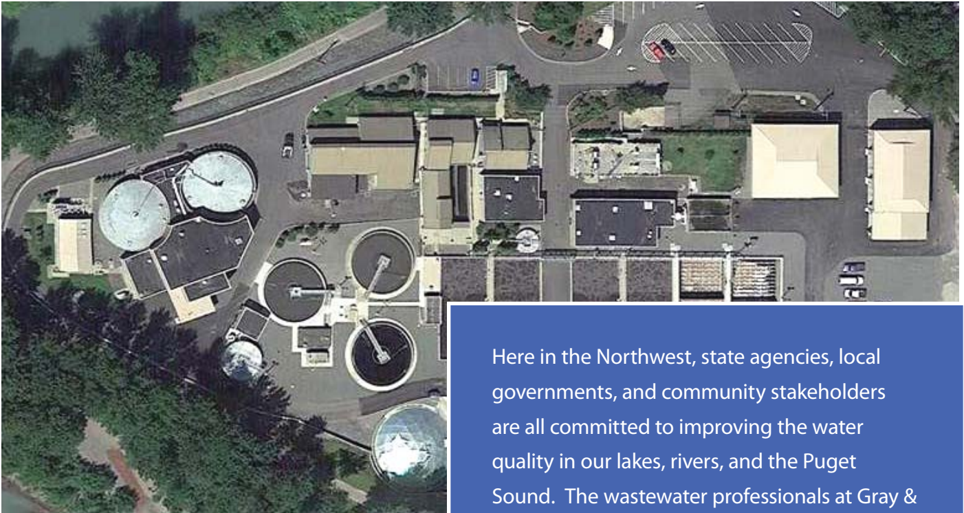
Sumner – Regional Wastewater Treatment Facility
