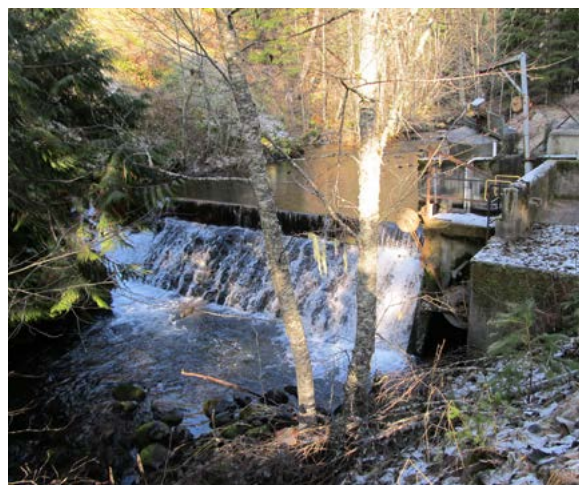
Buck Creek Diversion
