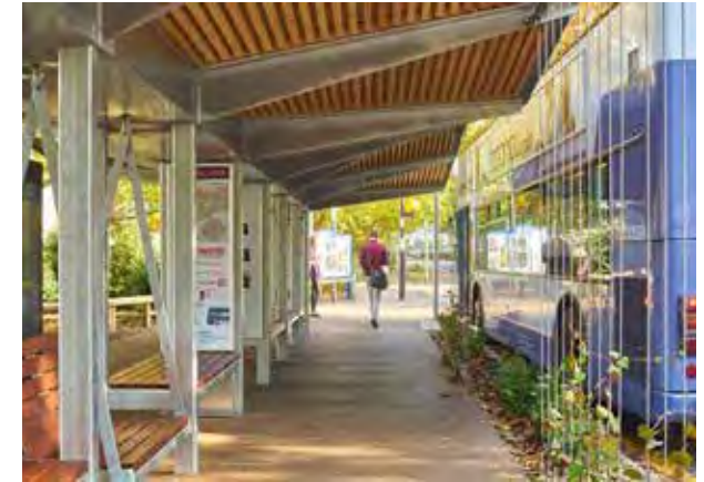
Shuttle shelter with signage and information.
