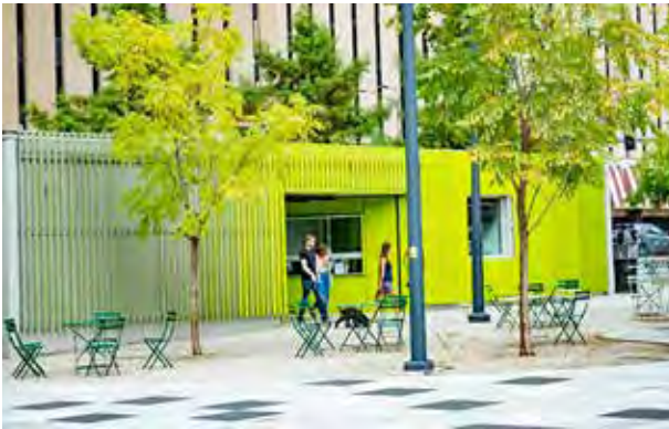
Small visitor contact facility with interpretive plaza.
