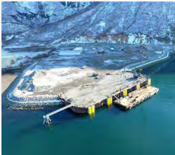
Sheetpile dock example (Chignik Public Dock)
