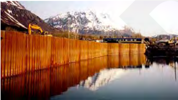
Sheet pile uplands expansion (Whittier and Seward)
