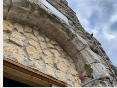
Archway Deterioration
