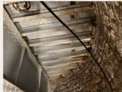
Corroded Steel
