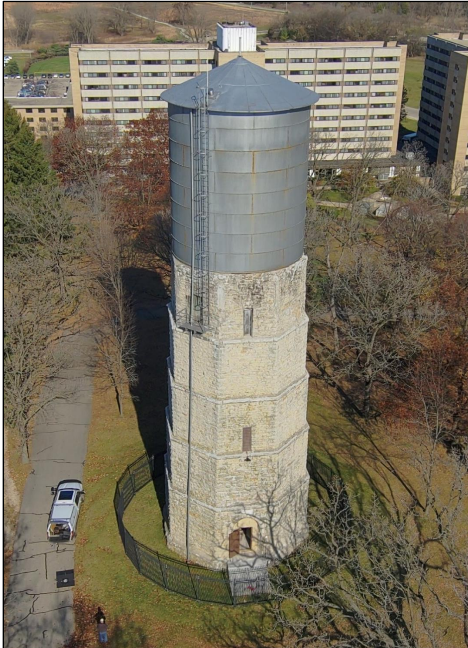
Photo 1: Starin Park Water Tower
