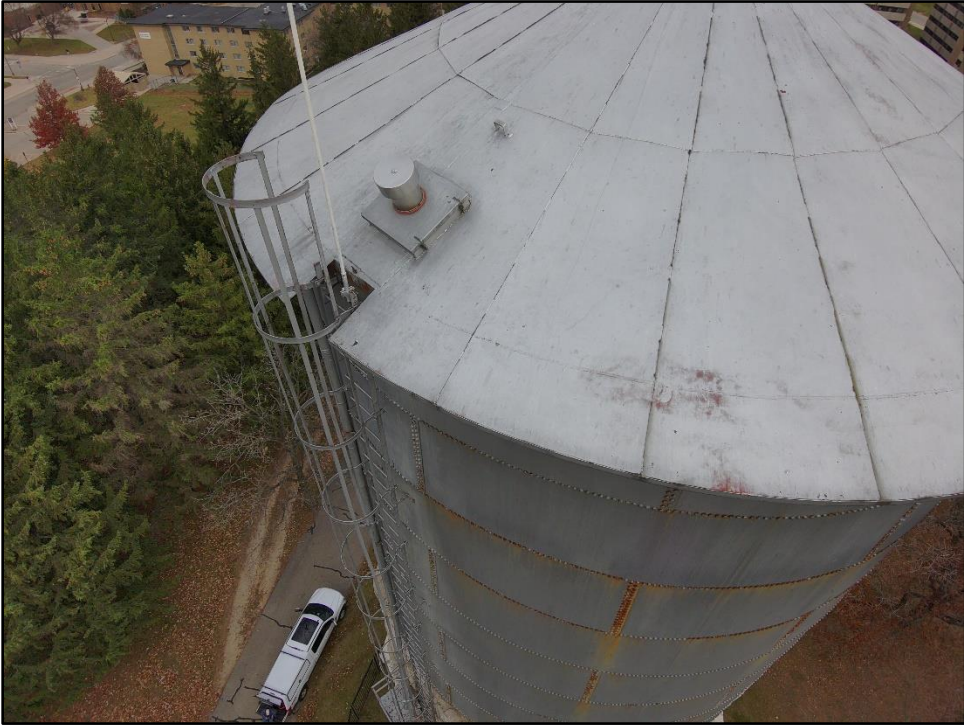
Photo 9: Exterior ladder to tank
