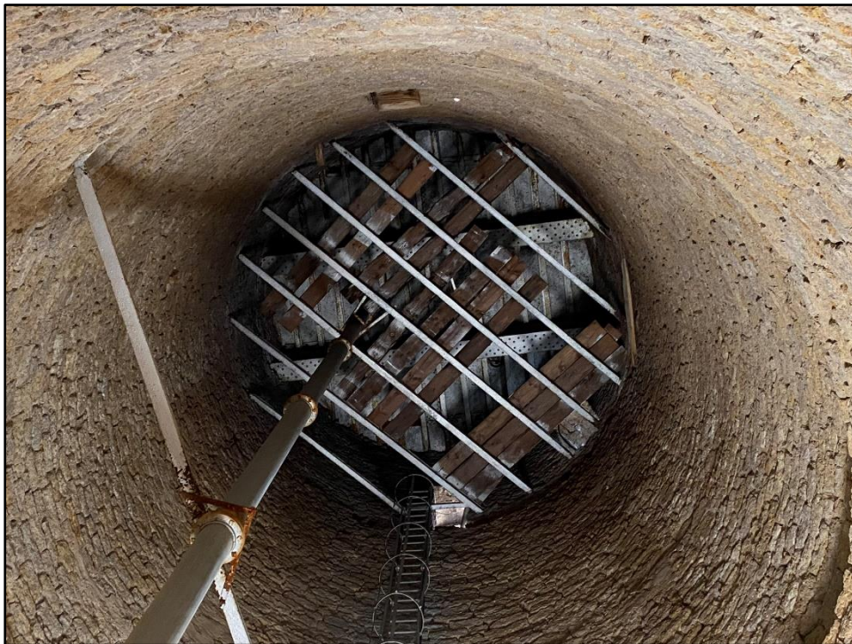
Photo 5: Floor and tank supports as viewed from below
