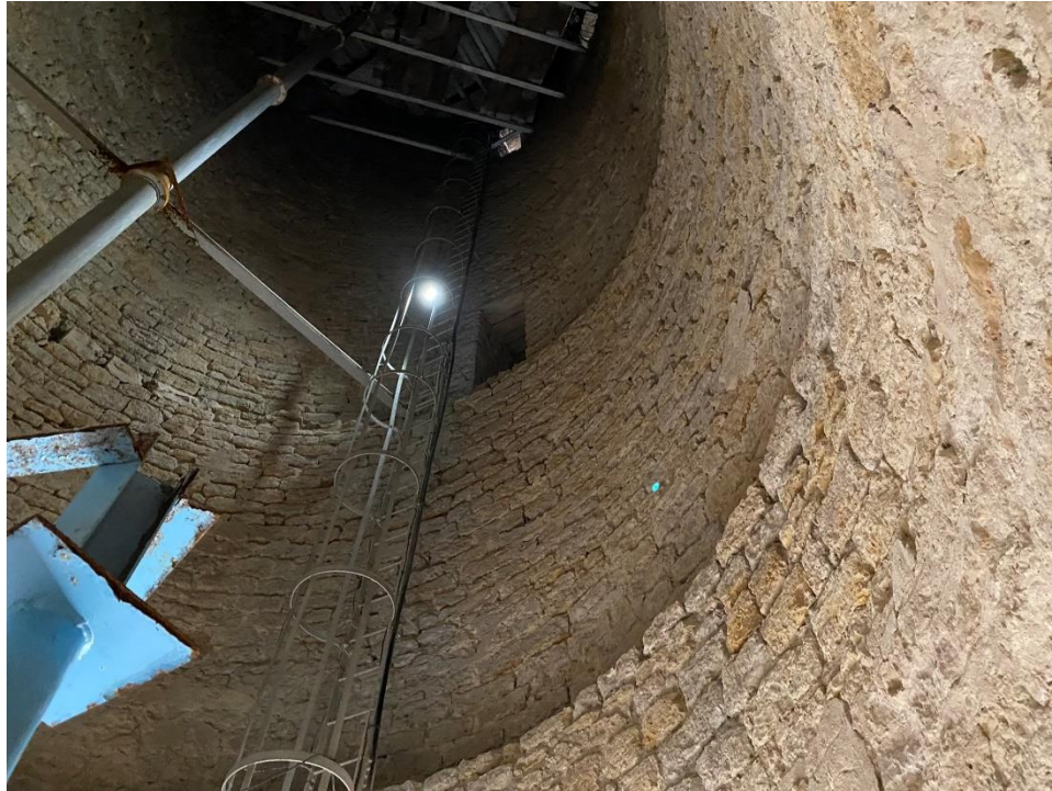
Photo 6: Ladder inside masonry tower
