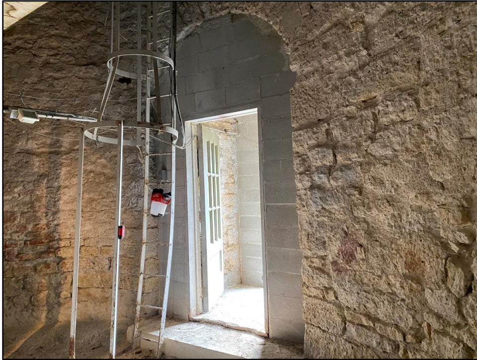
Photo 10: Modified entry door/wall
