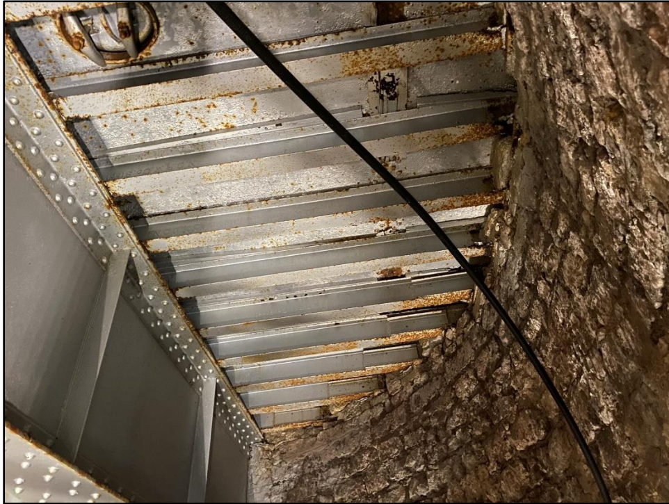
Photo 2: Steel beams below tank
