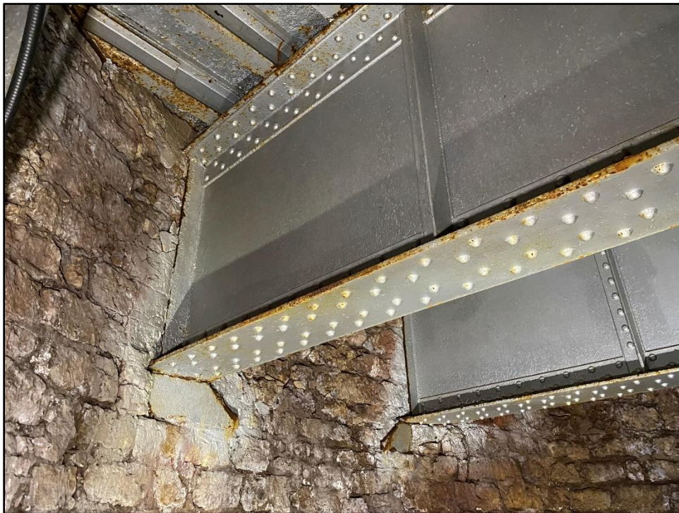
Photo 3: Steel plate girder supports
