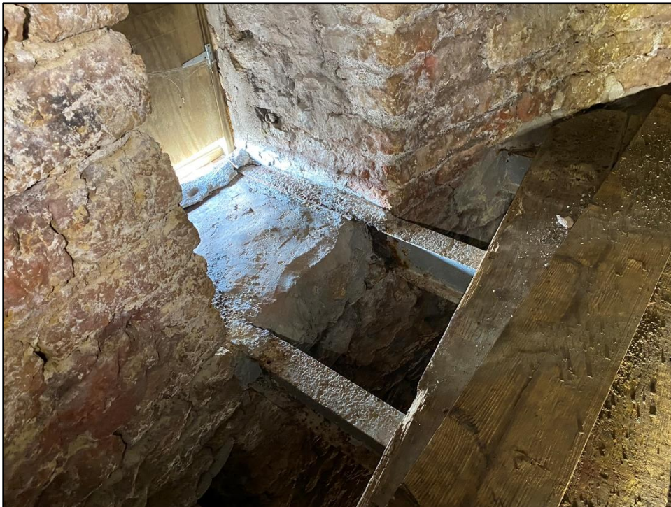
Photo 7: Doorway to exterior platform and ladder
