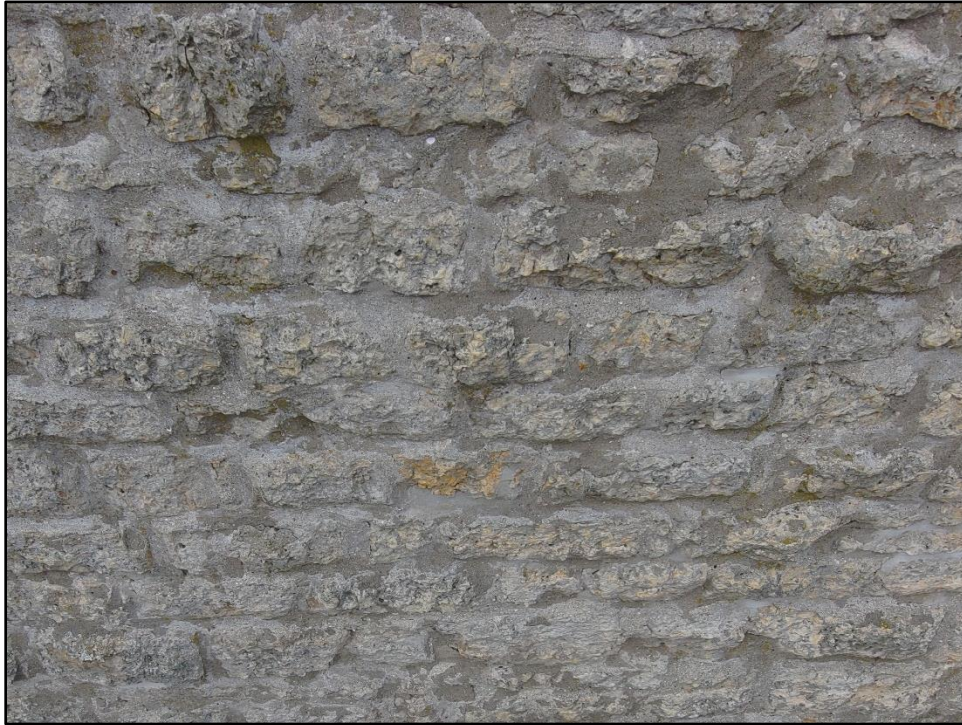
Photo 26: Repointed joints at mid-height of tower
