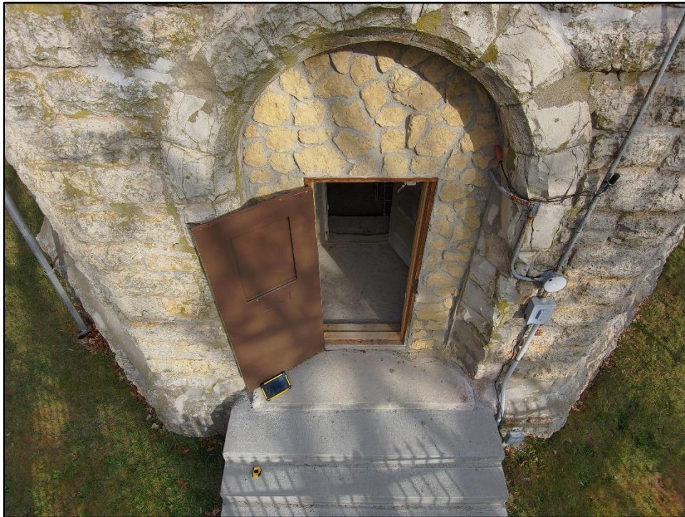
Photo 11: Modified entry door/wall
