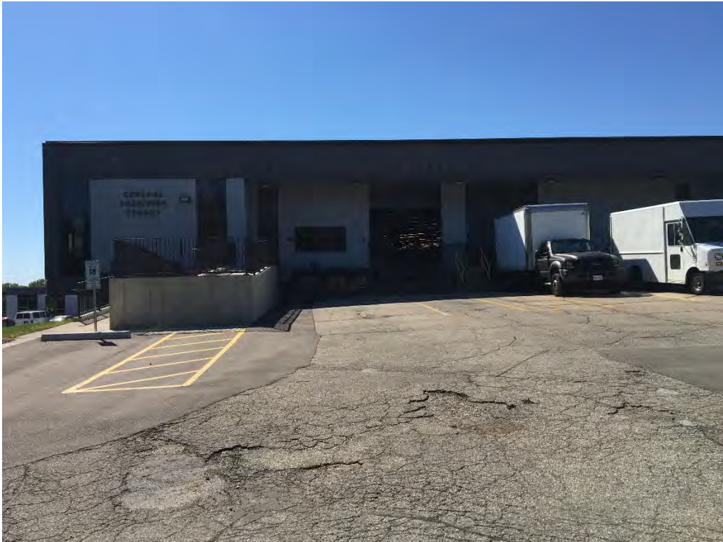
Looking South at General Services Building near winter salt brine equipment.
