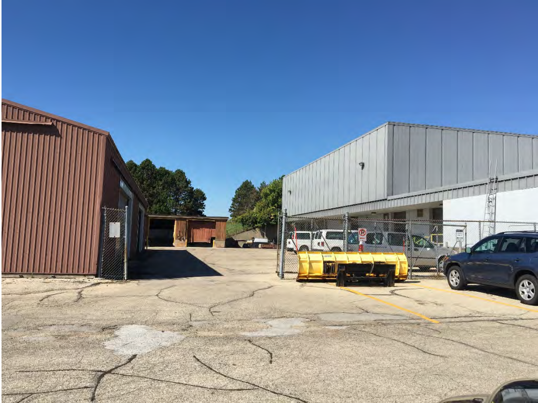
Looking West at south side of General Services Building.
