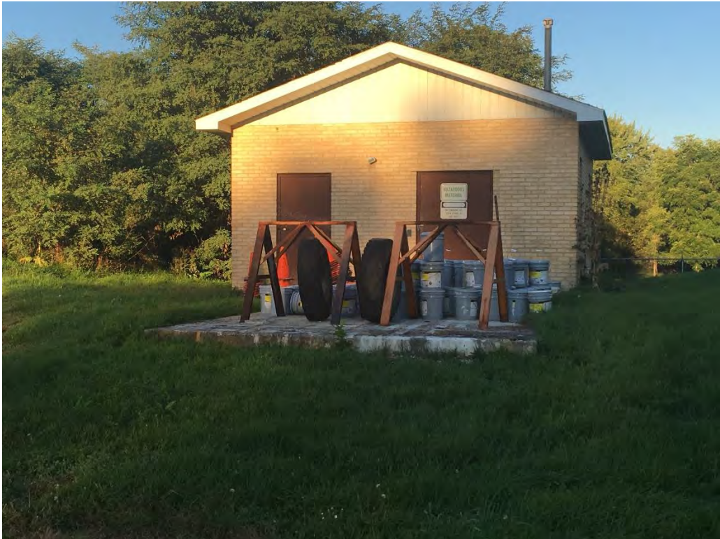
Looking west at Hazardous Material Storage Building
