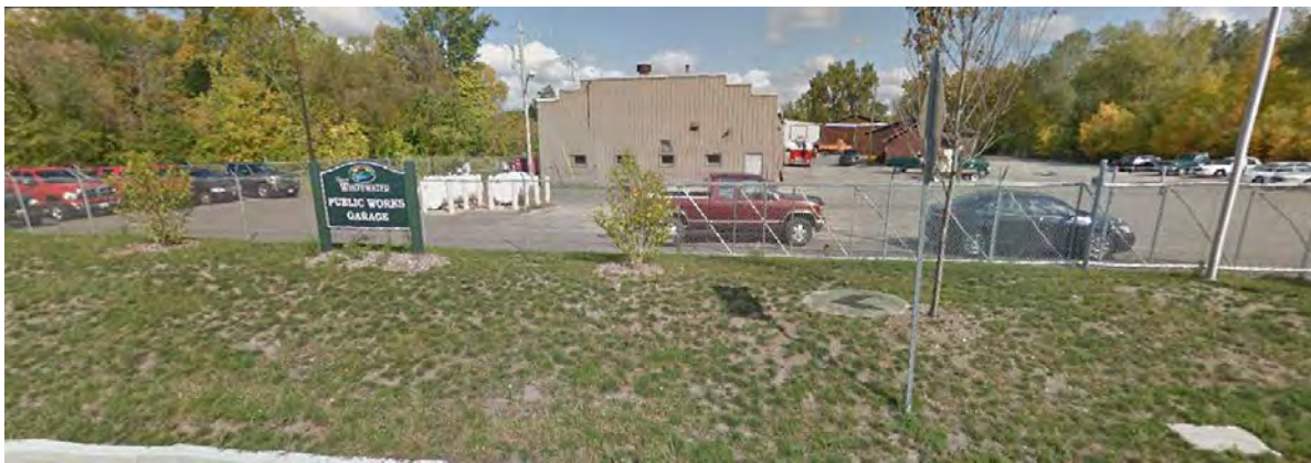
Figure 3.01-2 Public Works Garage (150 East Starin Road)
