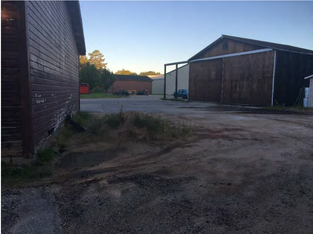
Looking Northwest at Salt Storage Building
