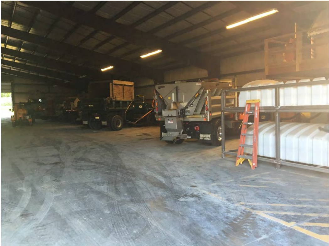
Looking Northeast in Cold Storage Building
