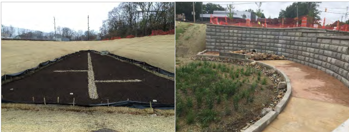
Figure 5.04-1 Enhanced Bioretention Basins in Cleveland, Ohio Serving 19-Acre and 59-Acre Drainage Areas, Respectively
