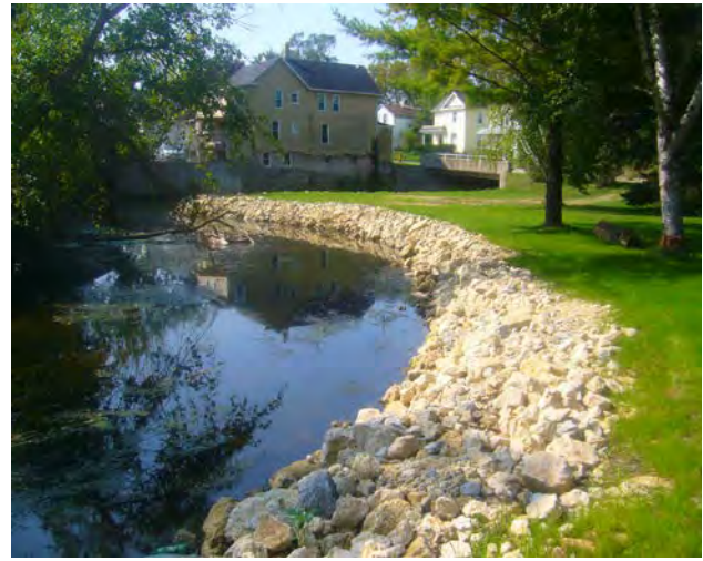
Figure 3.01-1 2015 Whitewater Creek Streambank Restoration
