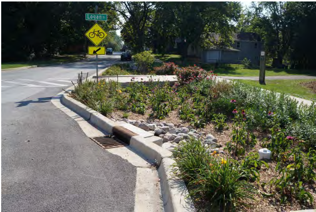
Figure 5.04-6 Traffic-Calming Bioretention Basin Bumpout System
