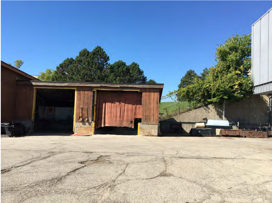
Looking west at salt storage shed.
