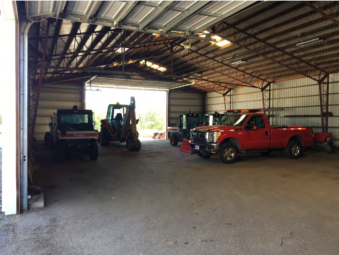
Looking Southeast at inside of cold storage building south of General Services Building.
