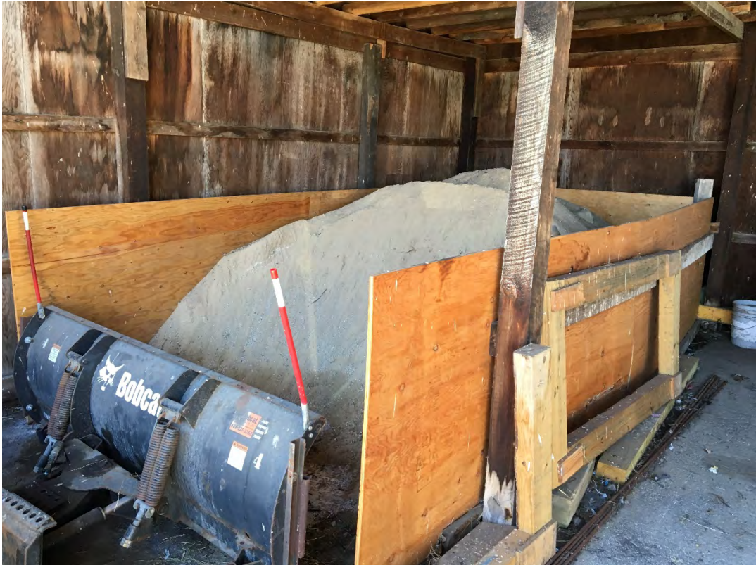
Looking Southwest at inside of sand storage shed.
