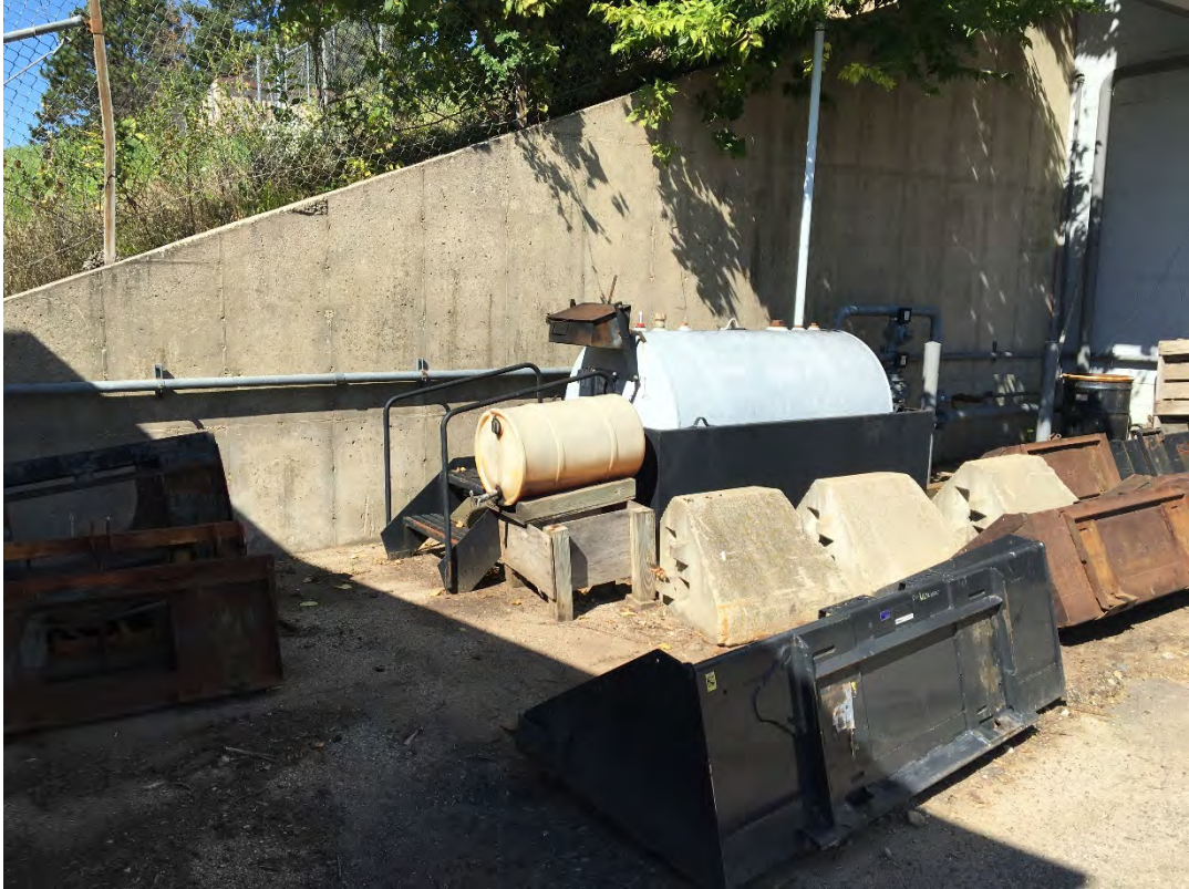
Looking Northwest at used oil storage tank.
