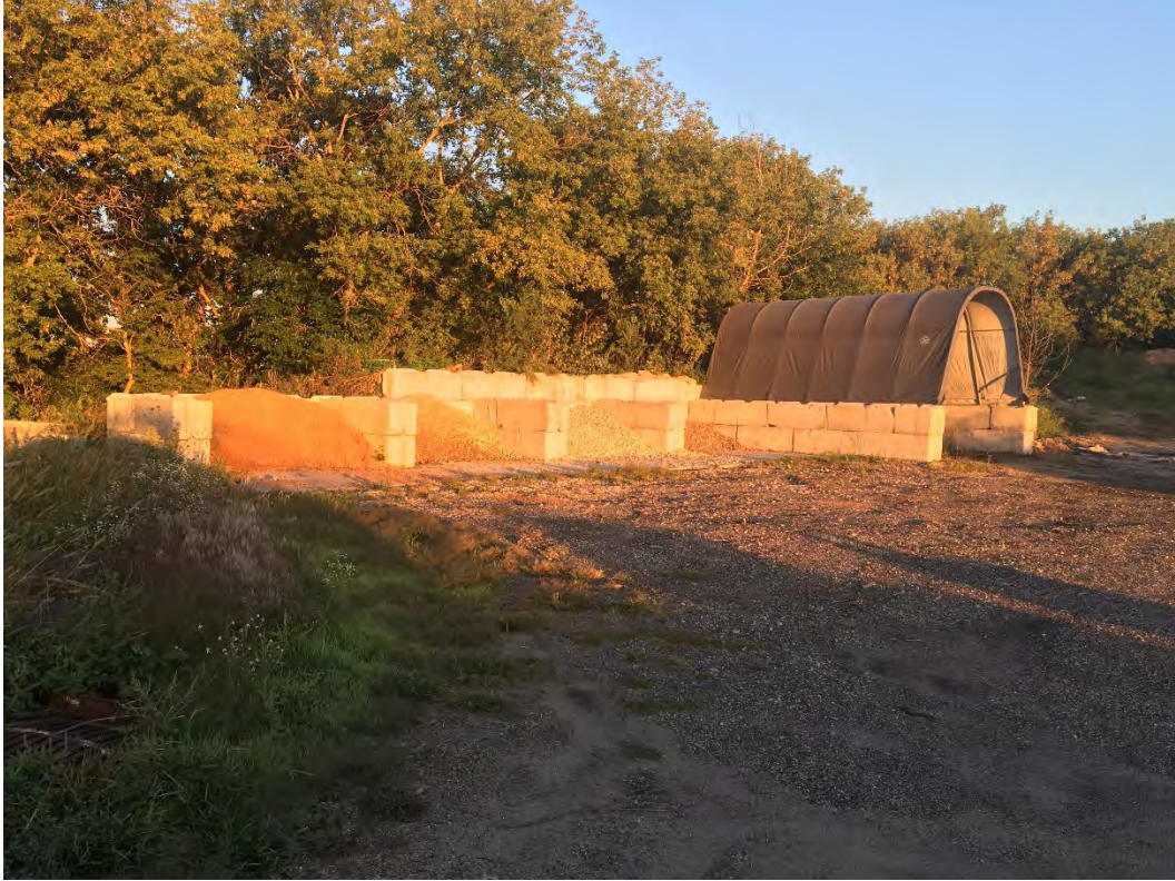
Looking Northwest at gravel storage areas.
