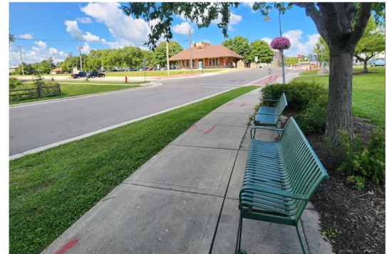
Fremont Street reconstruction project.
