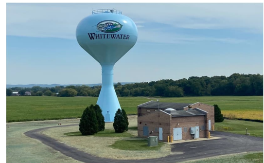
Well No. 9 and the Southwest Elevated Tank.
