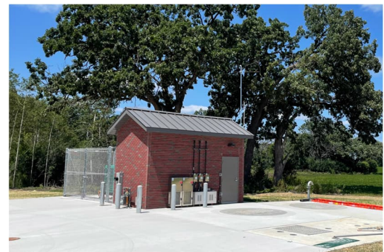
Vanderlip Pumping Station.
