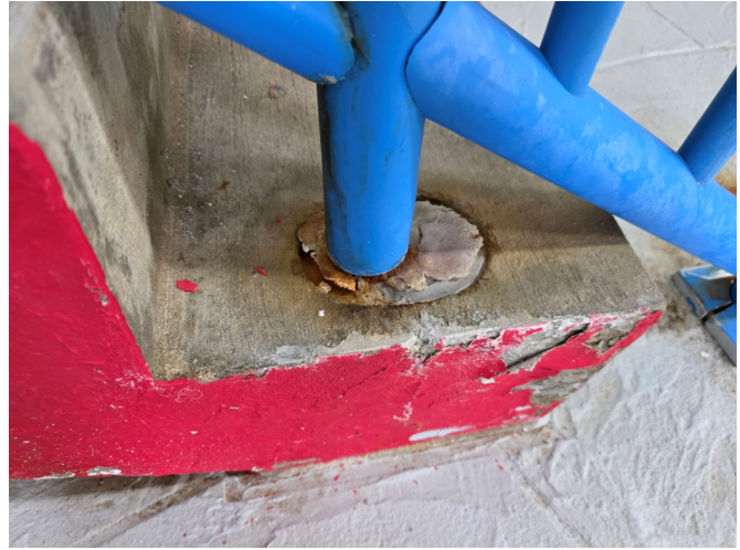
8. CRACKED/DETERIORATING CONCRETE
