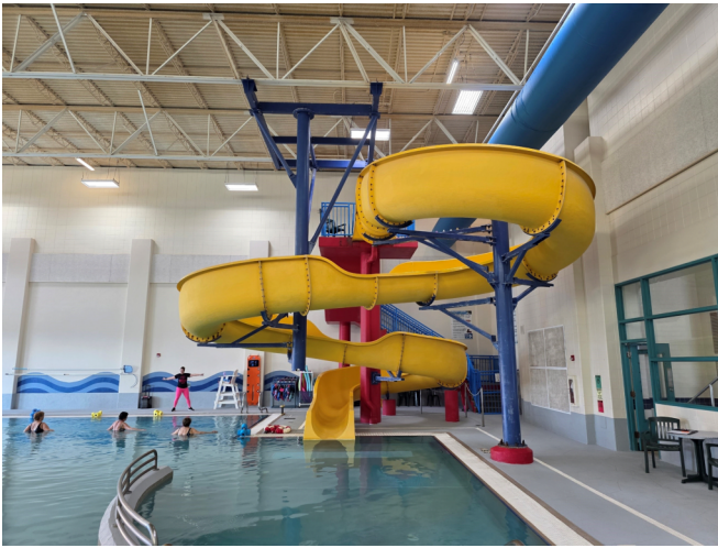
1. OVERALL VIEW OF THE SLIDE
