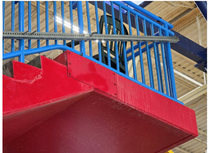
12. STRUT INSTALLED TO SUPPORT RAILINGS
