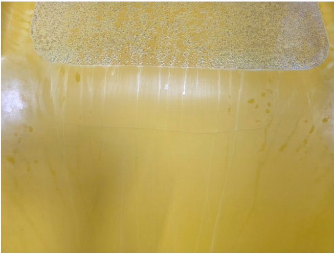
13. SCRATCH IN THE FLUME ENTRY TUB
