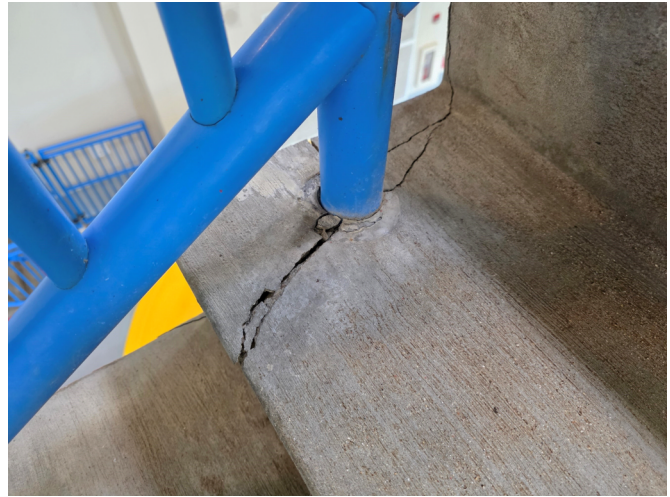
10. CRACKED/DETERIORATING CONCRETE
