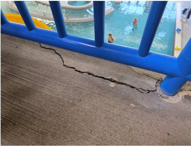
9. CRACKED/DETERIORATING CONCRETE
