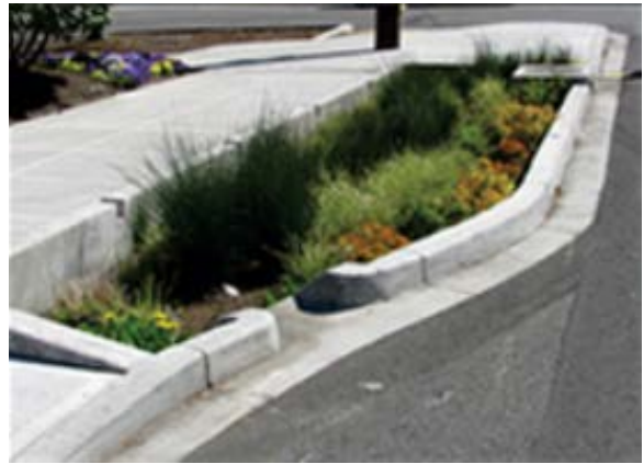
Figure 5: Example of a rain garden along rights-of-way
