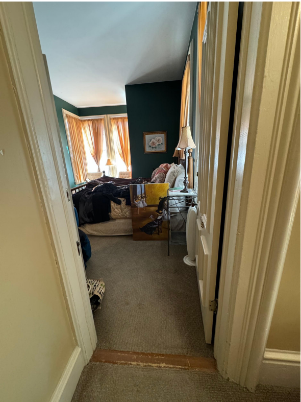
31 1/2" wide access to Monet suite for bathroom inside Need to review with city building inspector (1/2" to keep historic trim)
